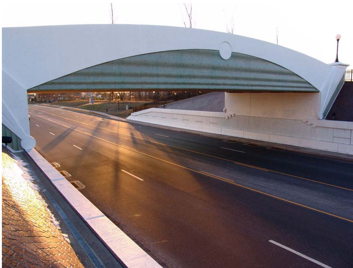
Figure 9 – The sloped walls above the MSE retaining walls reduced the sense of depth of the roadway and were constructed with standard concrete unit pavers and stabilized with geogrid reinforcement. The pavers were finished with dark mortar and urethane anti-graffiti treatment.
