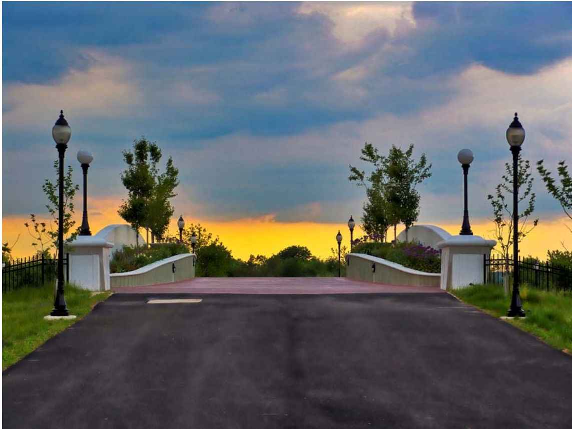
Figure 10 – The portal elevation of the bridge reveals the sweeping forms of the concrete landscape planters that echo the curves of the fascia beams and deck. The planters are insulated, waterproofed for drainage and automatic irrigation. Plant material was selected for harsh microclimate extremes.
