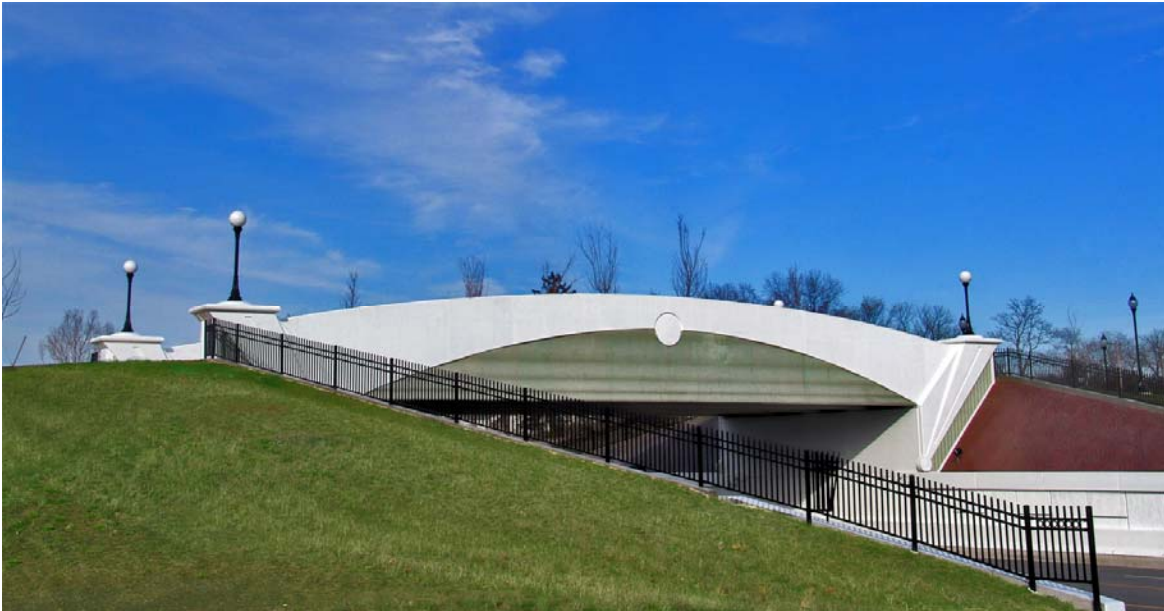
Figure 1 - Forty Foot Road Pedestrian Bridge is an 80-foot long by 40-foot wide, single span, signature bridge over a 5-lane Pennsylvania highway, and the featured centerpiece of a "context sensitive design" highway infrastructure project to create transportation improvements through a redeveloping town center. Completed in 2007.
