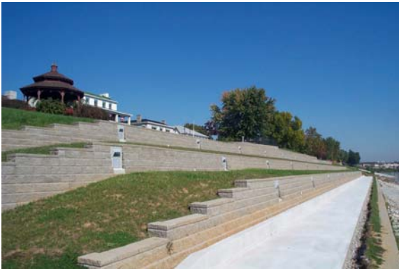
Fig. 10 Retaining Wall Terraces
