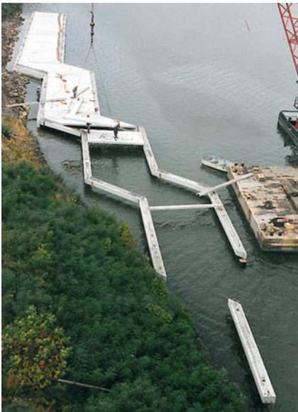
Fig. 4 Handicap Fishing Pier under Construction
