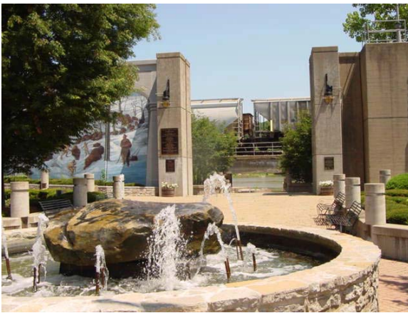
Fig. 2 Limestone Landing and Opening through Floodwall
