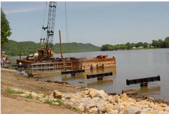
Fig. 7 Maysville Waterfront Expansion showing steel support cross-beams
