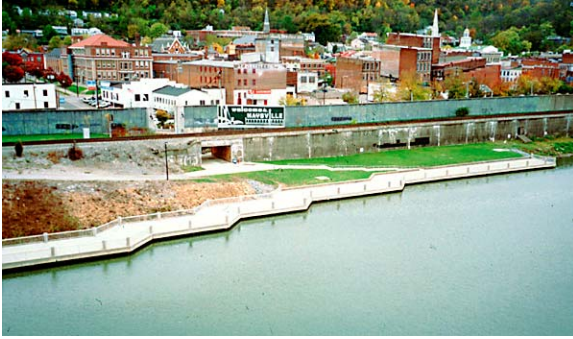
Fig. 5 Finished Handicap Fishing Pier
