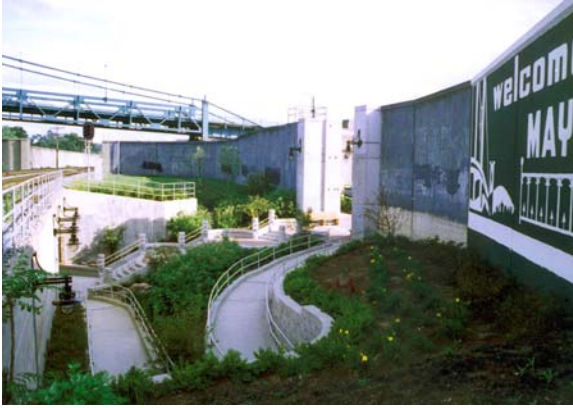
Fig. 3 Terraced Stair and ADA Compliant Ramp
