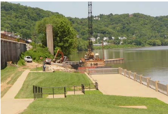
Fig. 6 Maysville Waterfront Expansion (currently under construction, July 2008)
