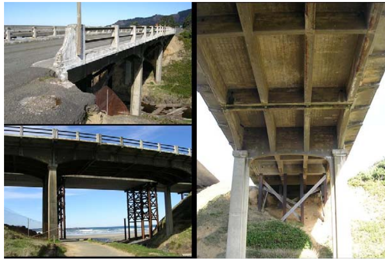
Fig. 1 – Existing Spencer Creek Bridge
