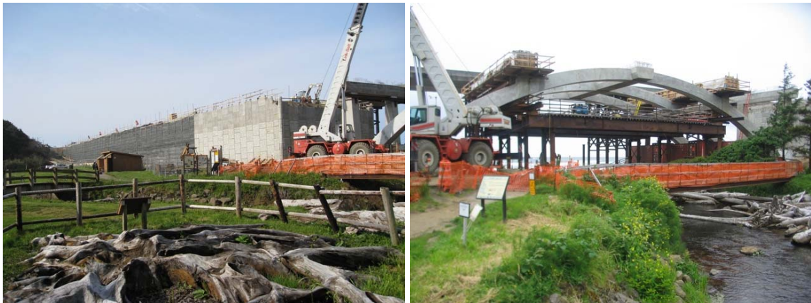
Fig. 8 – New Spencer Creek Bridge Construction
