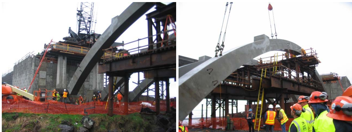
Fig. 5 – South-East Arch Rib Set
