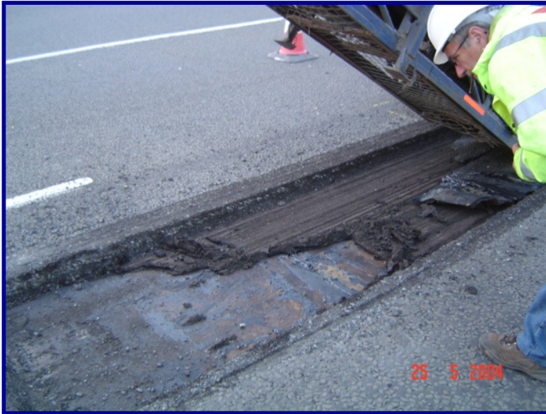
Planing trials removed the old sheet waterproofing membrane and revealed unbonded membrane with moisture present under bituminous sheet system
