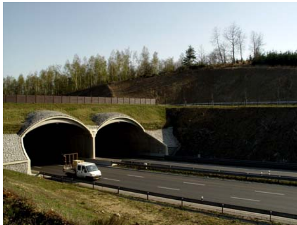
Fig. 3 Insensible earthworks at the ecological bridge near Drhovle
