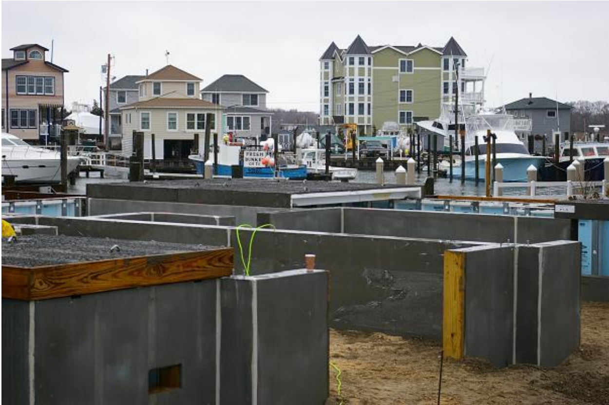
Fig. 4 The new precast floor panel system in place.
