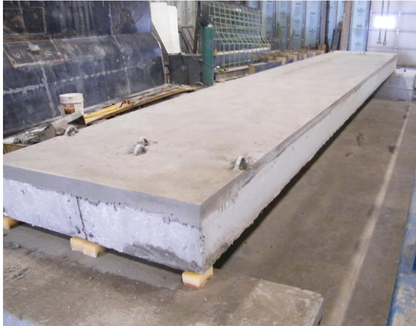
Fig. 10 Plank on urethane bearing pads
