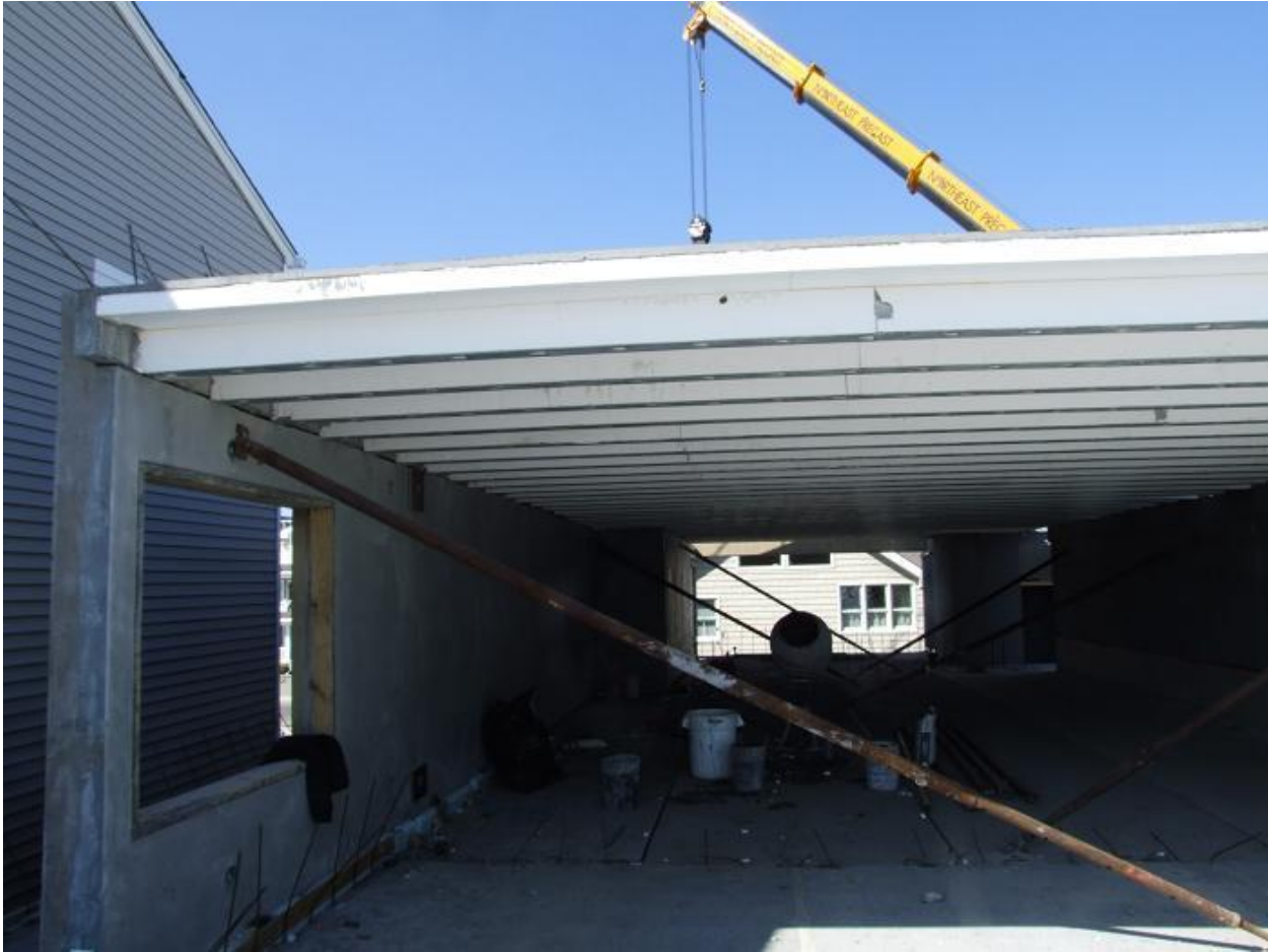
Fig. 2 The floor panels placed side by side on a bearing wall.
