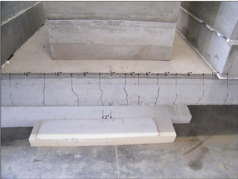
Fig. 14 Cracking at mid-span after step 8
