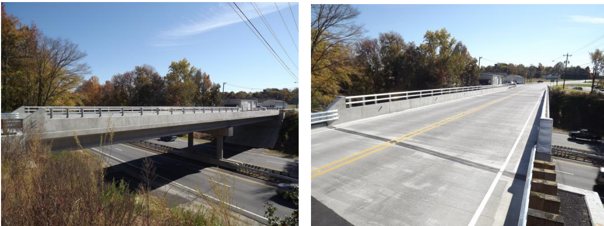
Figure 3 - Photos of Completed Bridge
