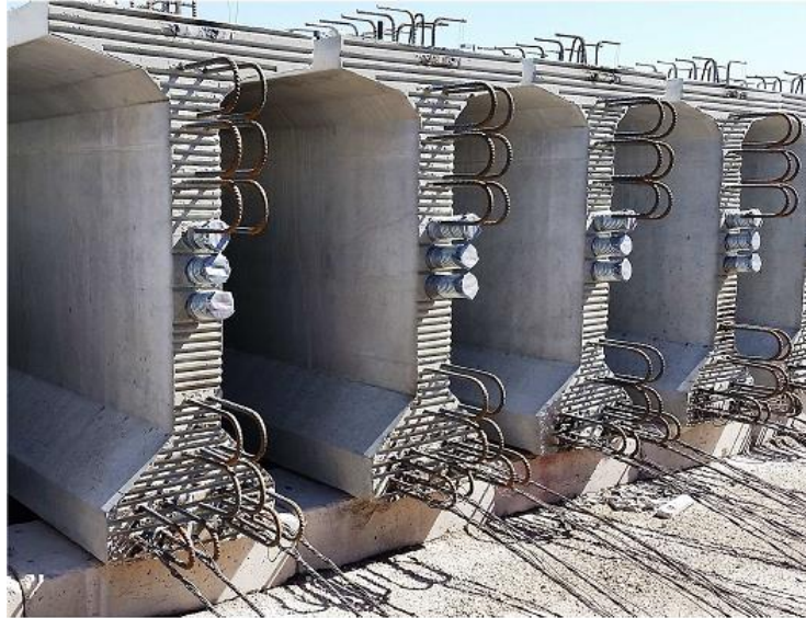
Figure 12 – PT Ducts and Precast Girder End Treatment
