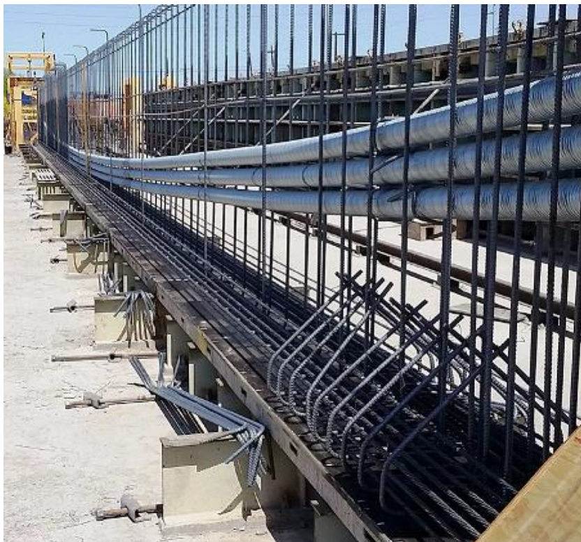
Figure 11 – PT Ducts in Precast Girder Web
