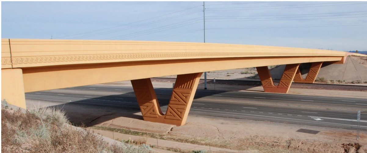
Figure 3 – Existing US60/SR303L Bridge
