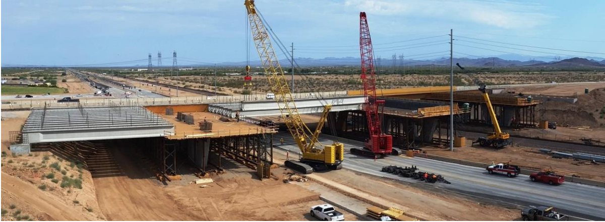
Figure 23 – Setting Girders at Span 2
