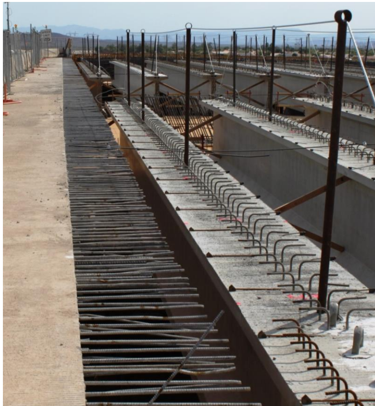
Figure 10 – Existing Reinforcing at Deck Closure Pour
