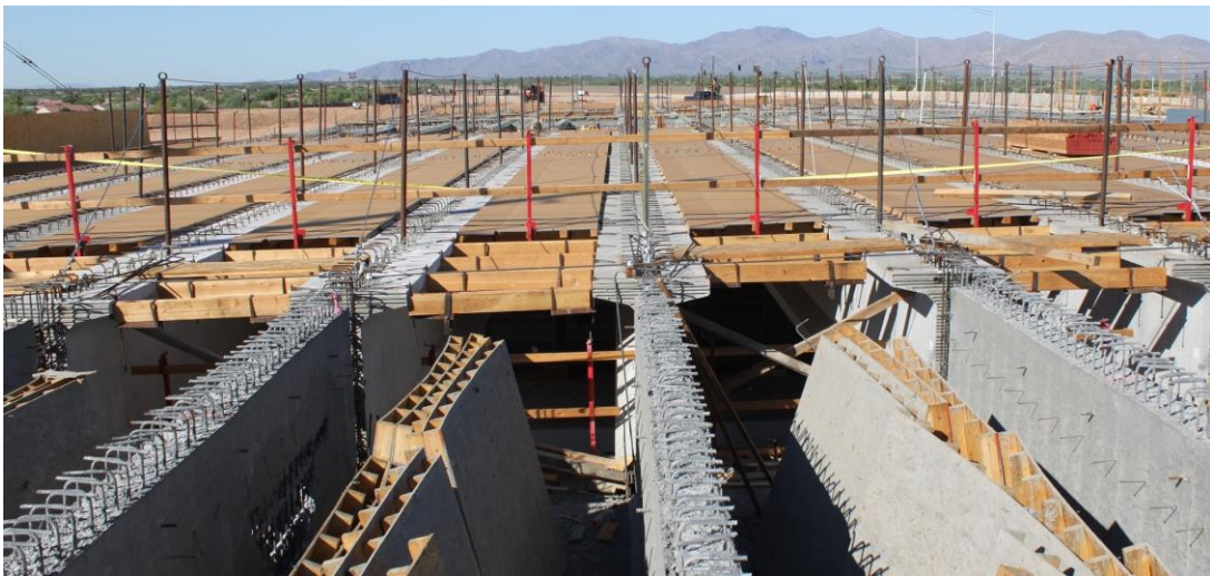
Figure 13 – Girder Lines at CIP Webs & Precast Girders
