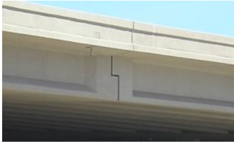
Figure 19 – Photo of Similar Completed Hinge
