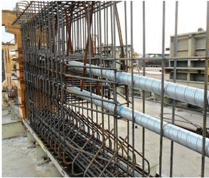
Figure 15 – PT Ducts and Reinforcing at Precast (Photo by Jason Kuck, Tpac)
