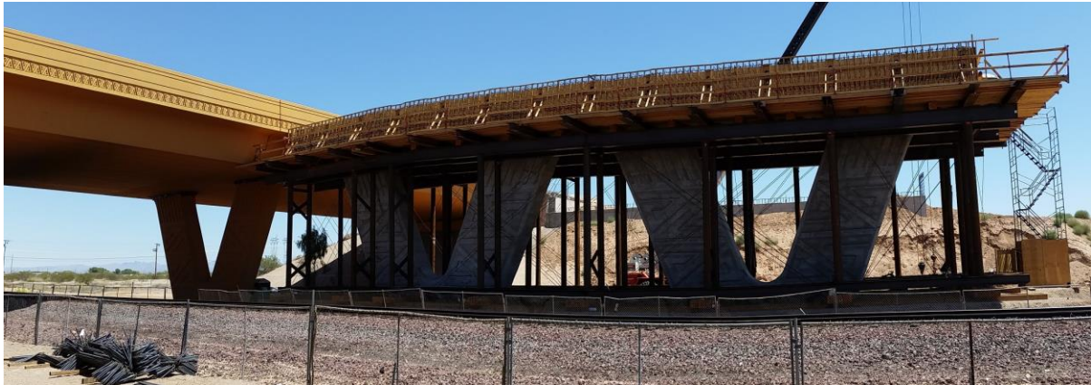
Figure 17 – Elevation Pier 3 at Drop-In Span
