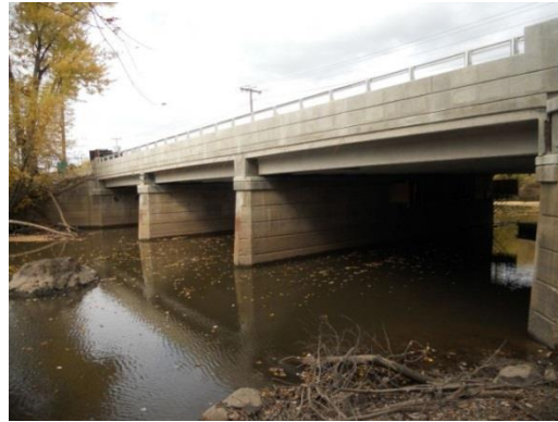
Photo 11 – Elevation view of the bridge with new superstructure.
