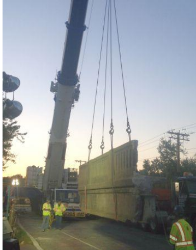
Photo 6 - Removal of fascia stringer and parapet.
