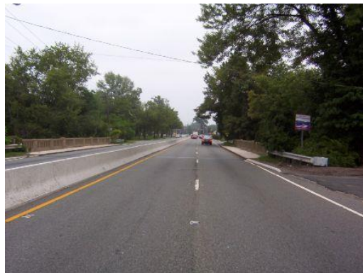
Photo 1 - West approach roadway, eastbound lanes, looking east.
