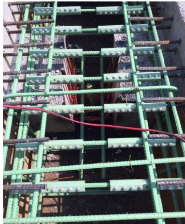
Photo 9 - Live load continuity pour couplers over pier (between bridge units).
