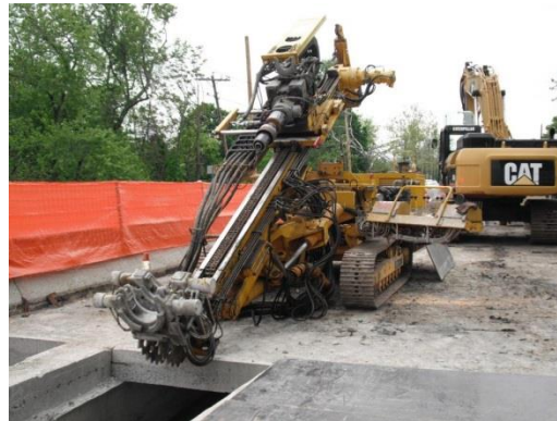
Photo 5 - Ground anchor installation through hole in concrete deck.
