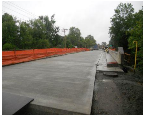
Photo 10 - Stage 1 HES concrete overlay on precast approach slabs and NEXT
