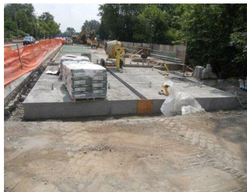
Photo 7 - Precast approach slabs ready for HPC closure pour.
