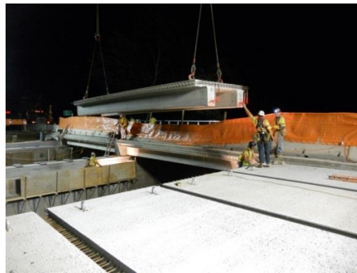
Photo 8 - Installation of prefabricated bridge unit.
