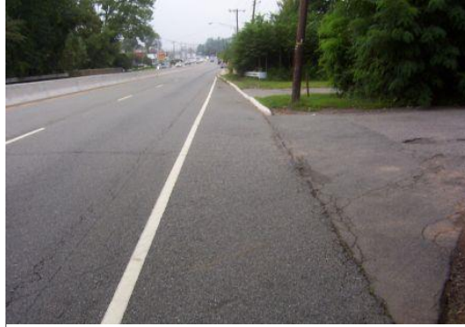
Photo 4 - Typical driveways adjacent to bridge within work zone.
