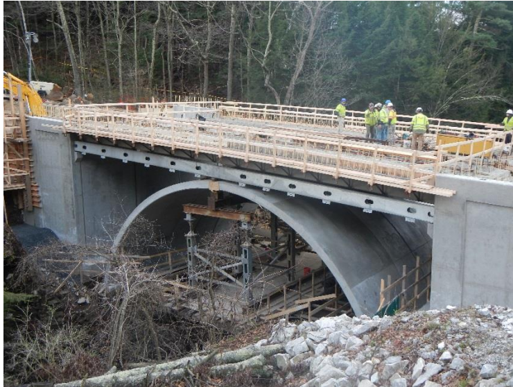
Figure 7: Bridge Elevation – Prior to Hanging Face Panels
