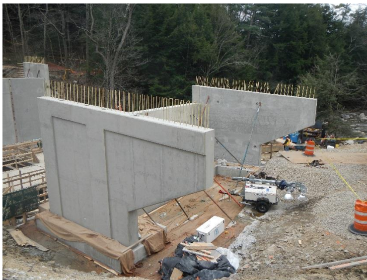
Figure 5: One Piece Precast Wingwalls 26' Long x 15' Tall
