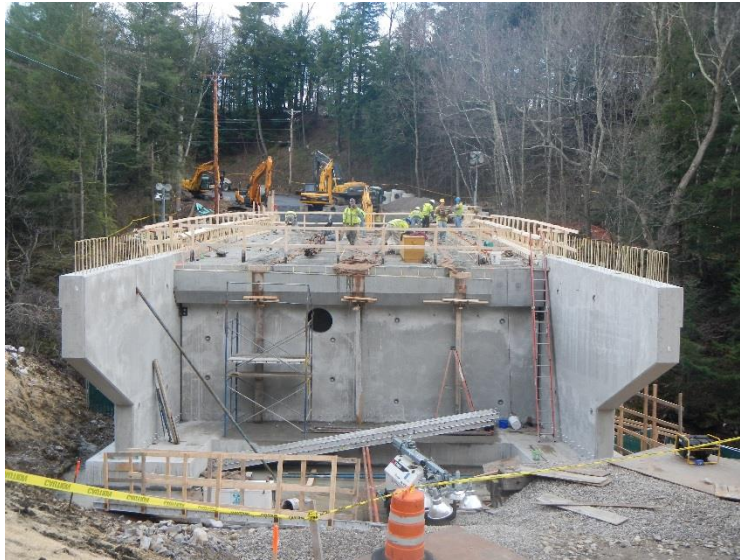
Figure 6: Abutments and NEXT Beams – Note Precast Curtain Wall
