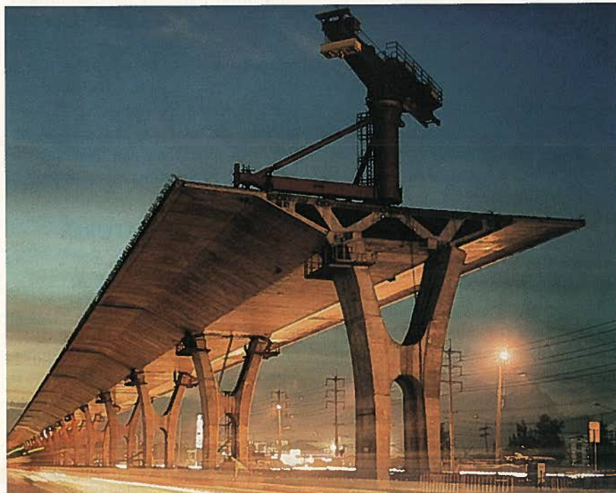
Fig. 3. Main line span of 44.40 m (146 ft).
