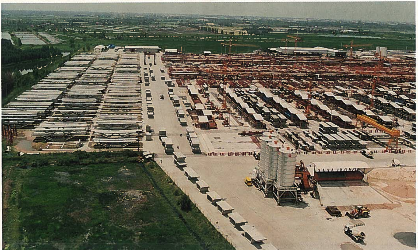
Fig. 13. Layout of precasting yard.
