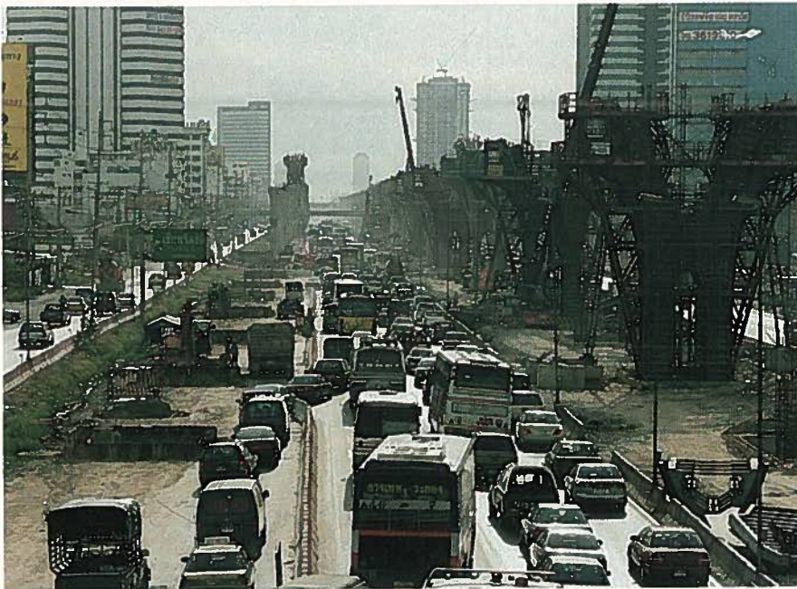
Fig. 2. Construction of the BNE project above congested Highway 34.
