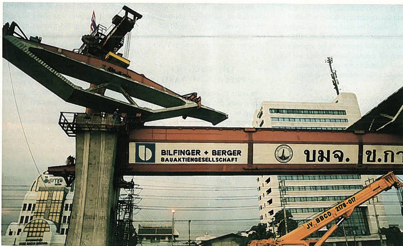
Fig. 12. Underslung erection girder.
