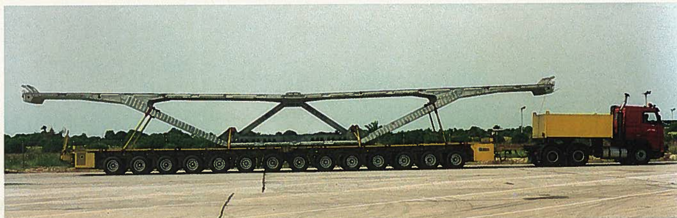
Fig. 16. D6 segment ready for transportation.
