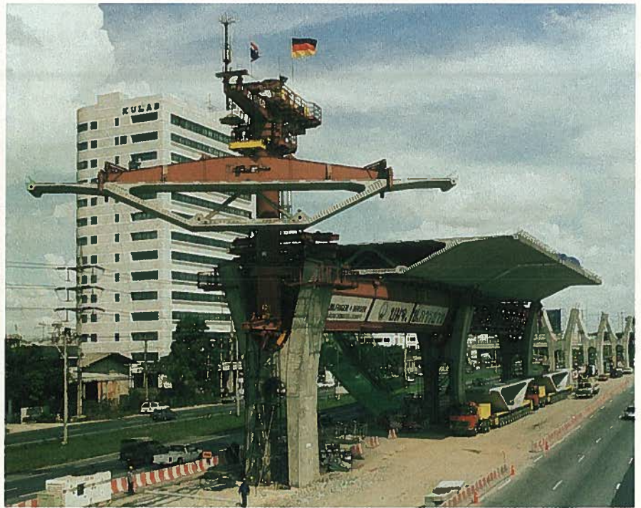
Fig. 17. Positioning of Segment D6 on mainline column.
