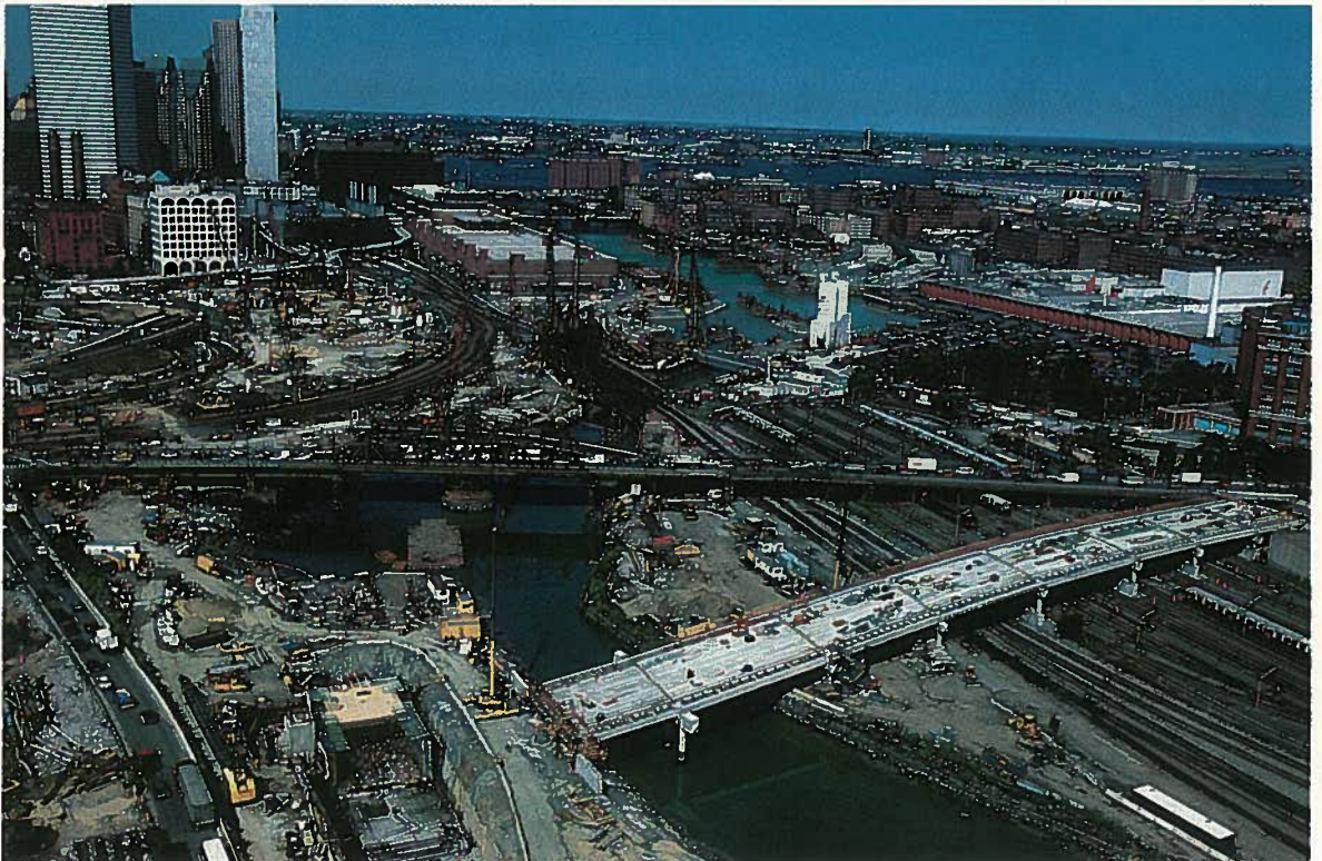
Fig. 4. Broadway Bridge under construction.
