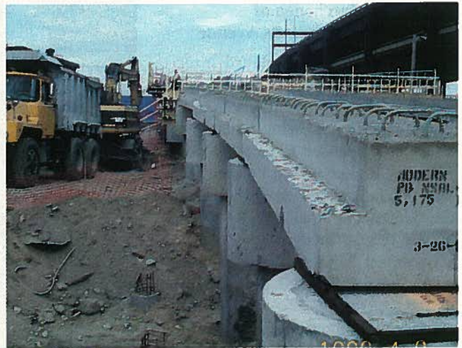
Fig. 6. Slab-on-pile construction.
