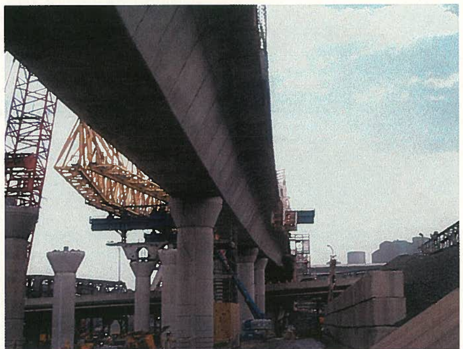
Fig. 11. Segmental concrete bridge erection.
