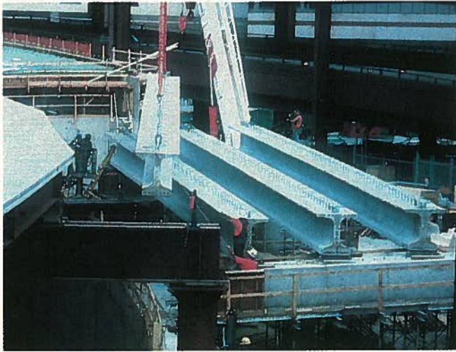
Fig. 5. New England bulb-tee girder installation.
