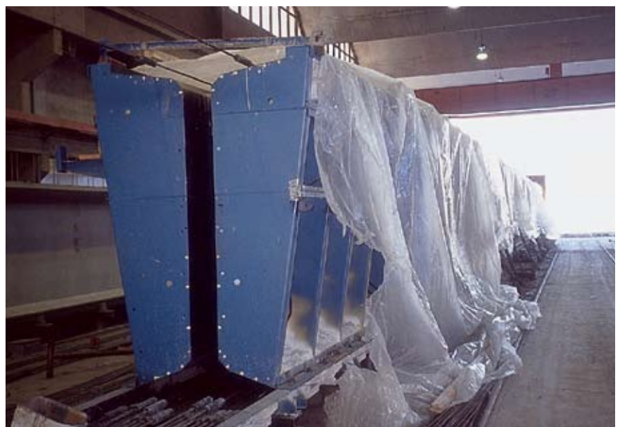
Fig. 10. Forms were installed with a visqueen moisture barrier.
