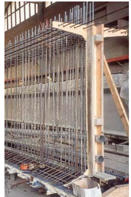
Fig. 9. Setup of middle girder segment.
