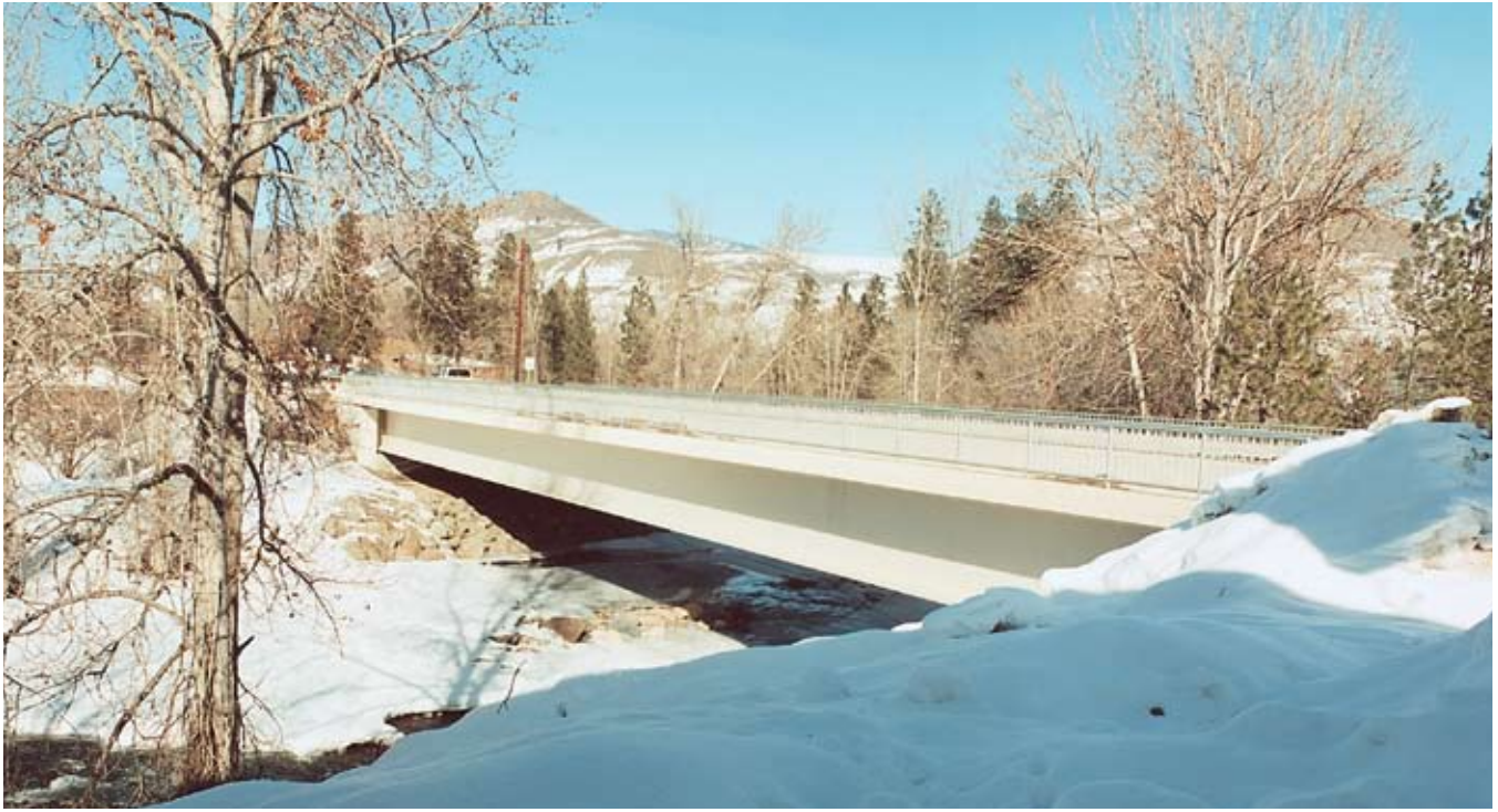
Fig. 20. Finished view of Twisp River Bridge (picture taken in February 2002). Courtesy: Alex Young, WSDOT Bridge Architect.
