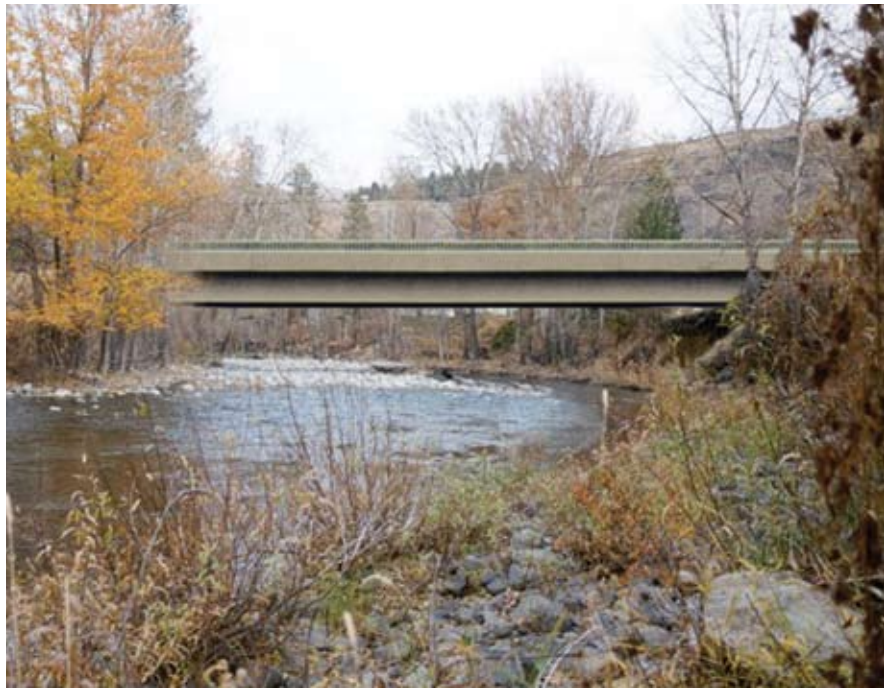
Fig. 17. Completed bridge in the fall of 2001.
