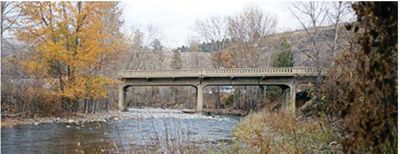
Fig. 4. Obsolete cast-in-place reinforced concrete T-beam bridge.
