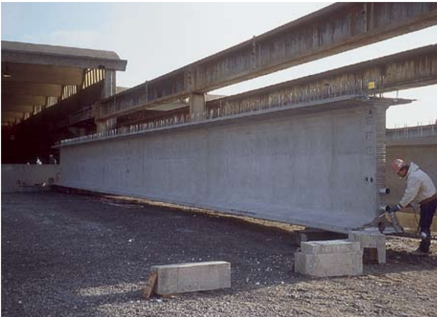
Fig. 11. Completed middle segment.
