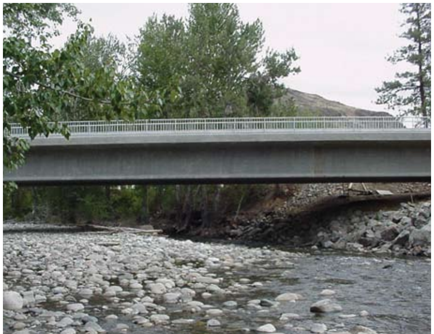
Fig. 18. Closeup of completed bridge.
