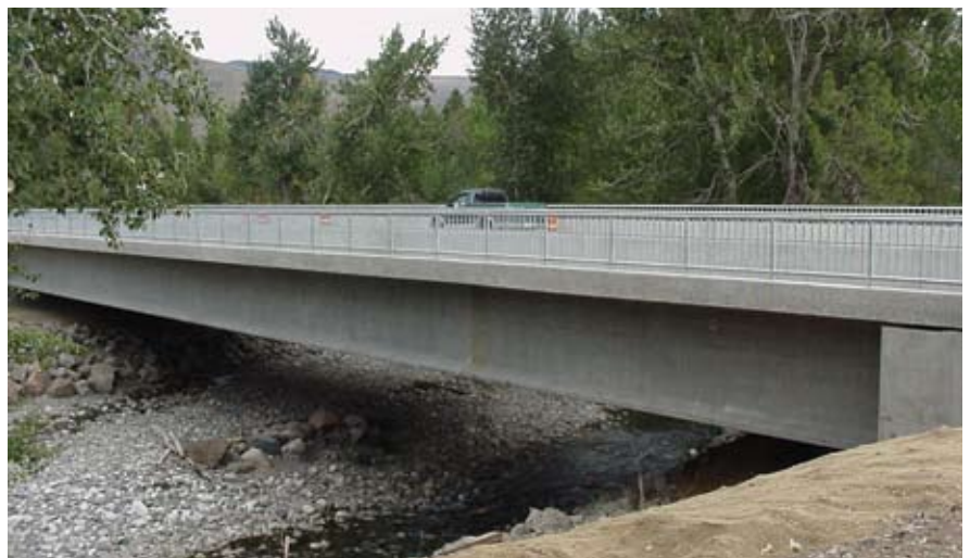
Fig. 2. Closeup of bridge showing new 2.4 m (7.87 ft) deep, W95PTMG girder.
