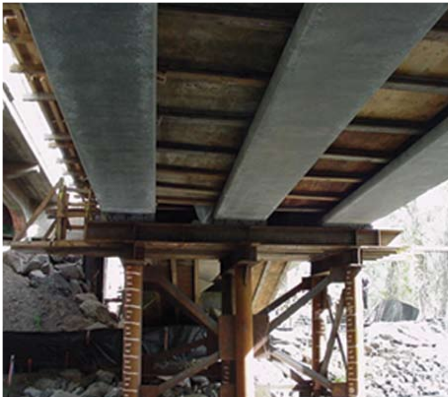
Fig. 14. Girder segments sitting on temporary falsework bents.
