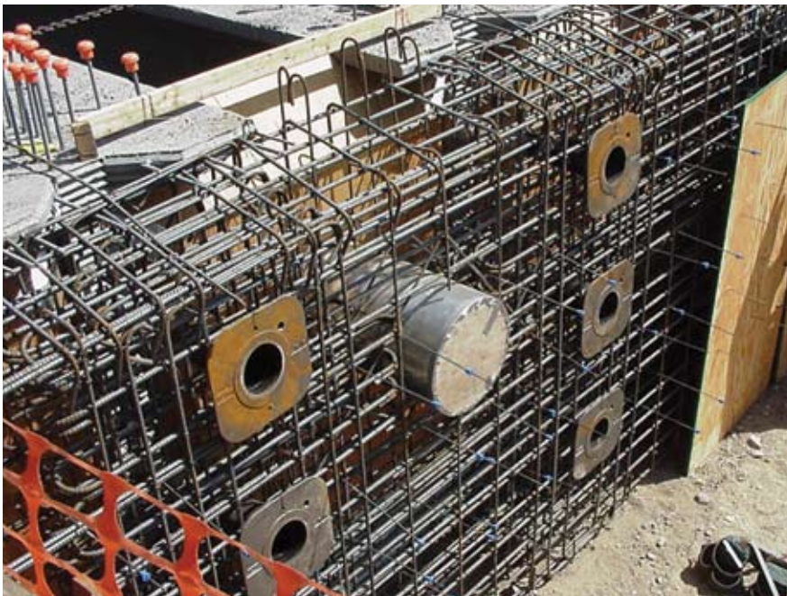
Fig. 8. Reinforcement and post-tensioning anchorages at end diaphragm.
