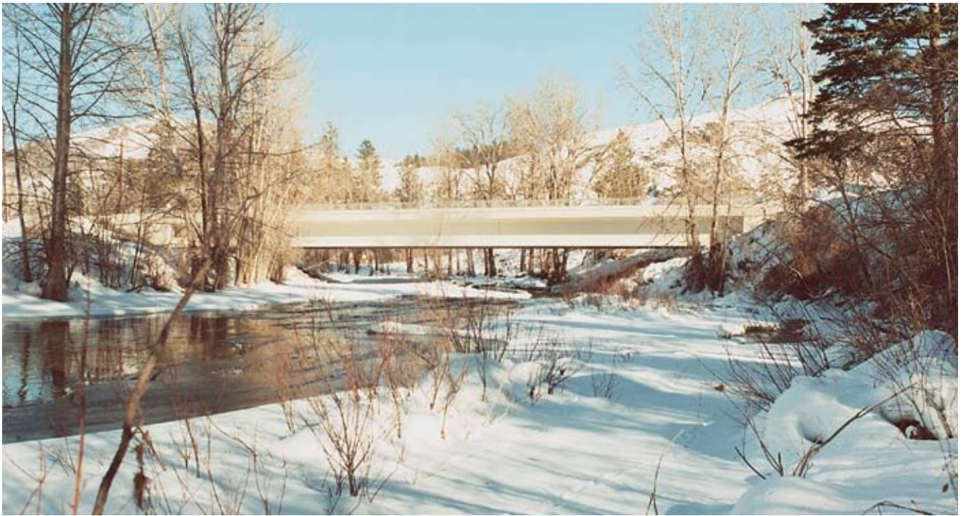
Fig. 1. Panoramic view of the Twisp River Bridge, Okanagon County, Washington State (picture taken in February 2002). Courtesy: Alex Young, WSDOT Bridge Architect.
