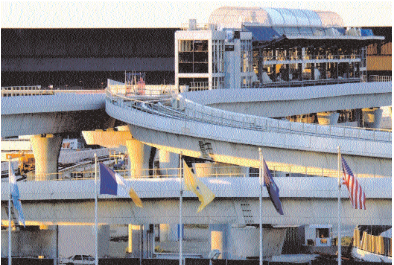
Fig. 18. The AirTrain Light Rail System was officially dedicated and opened to the public on December 17, 2003. Photo courtesy: Figg Engineering Group.
