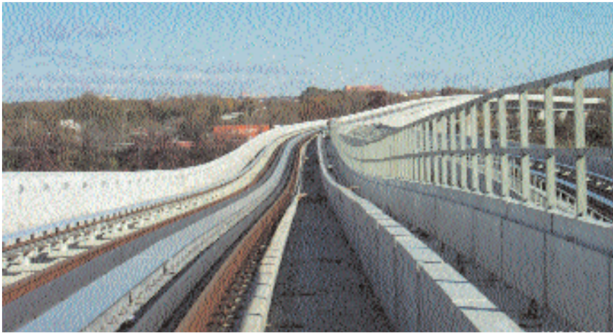
Fig. 8. Precast concrete side parapets functioned in dampening sound to the surrounding neighborhoods as well as concealing the track. Photo courtesy: Bayshore Concrete Products.
