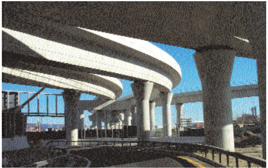
Fig. 6. The seamless transition and sleek line of the precast concrete superstructure is apparent in this ground shot. The beauty and elegance of the precast concrete design overcame over 30 years of public opposition to a light rail transit project. Photo courtesy: Bayshore Concrete Products.
