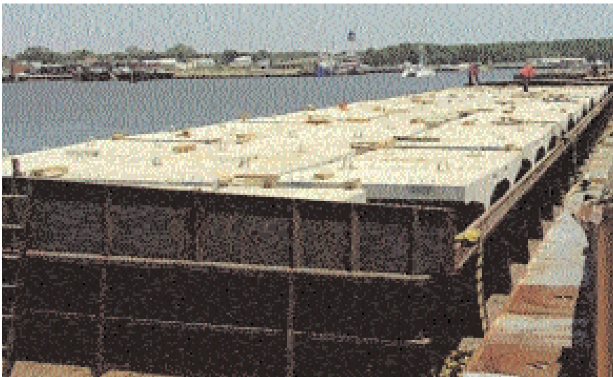
Fig. 14. On average, one loaded barge per week left the precast facility carrying approximately one week's production of segments. Photo courtesy: Bayshore Concrete Products.
