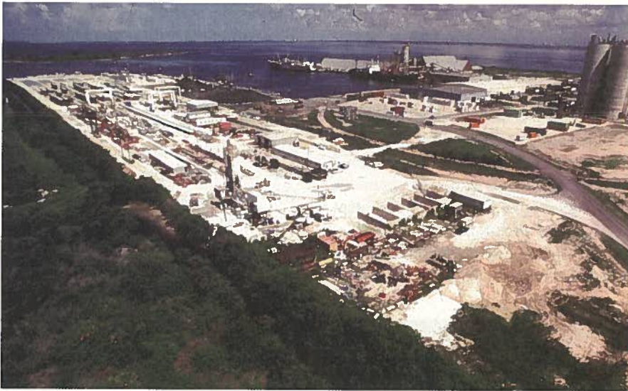
Fig. 18. Shown is the Sunshine Skyway Bridge precasting yard at Port Manatee, Fla.
