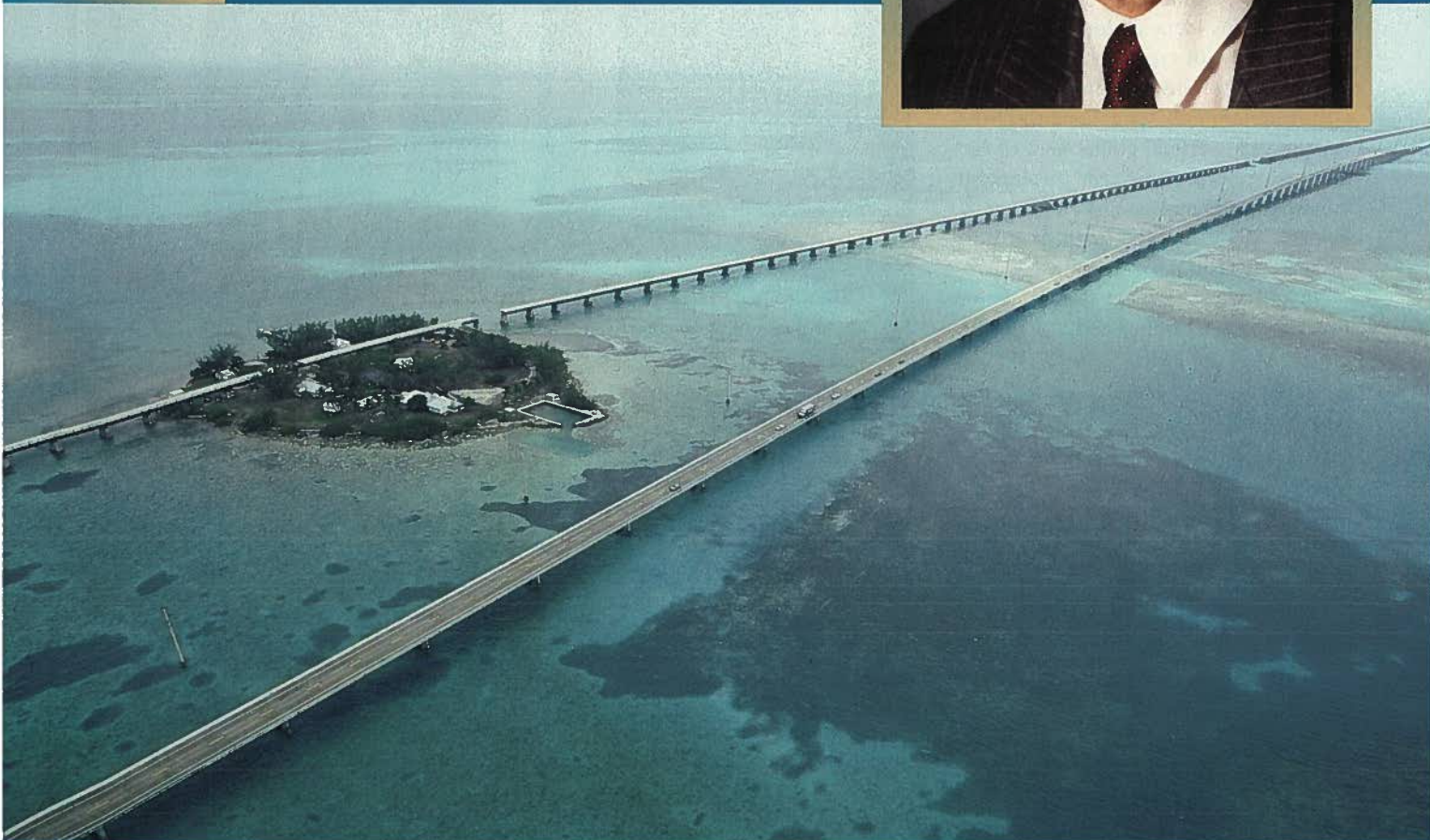
Fig. 14. Shown is the Seven-Mile Bridge in the Florida Keys. Photo courtesy of Figg & Muller Engineers.
