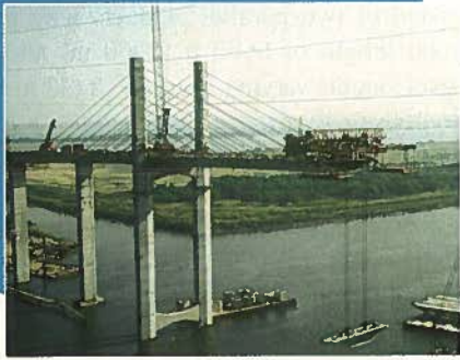
Fig. 21. Shown is the Neches River Bridge deck erection in Texas.
