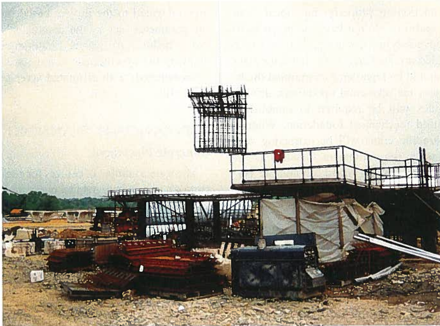
Fig. 3. Reinforcement jigs produce daily reinforcing steel cages.
