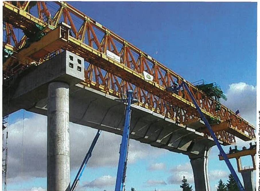
Fig. 11. Span-by-span precast concrete segmental construction using a launching gantry.
