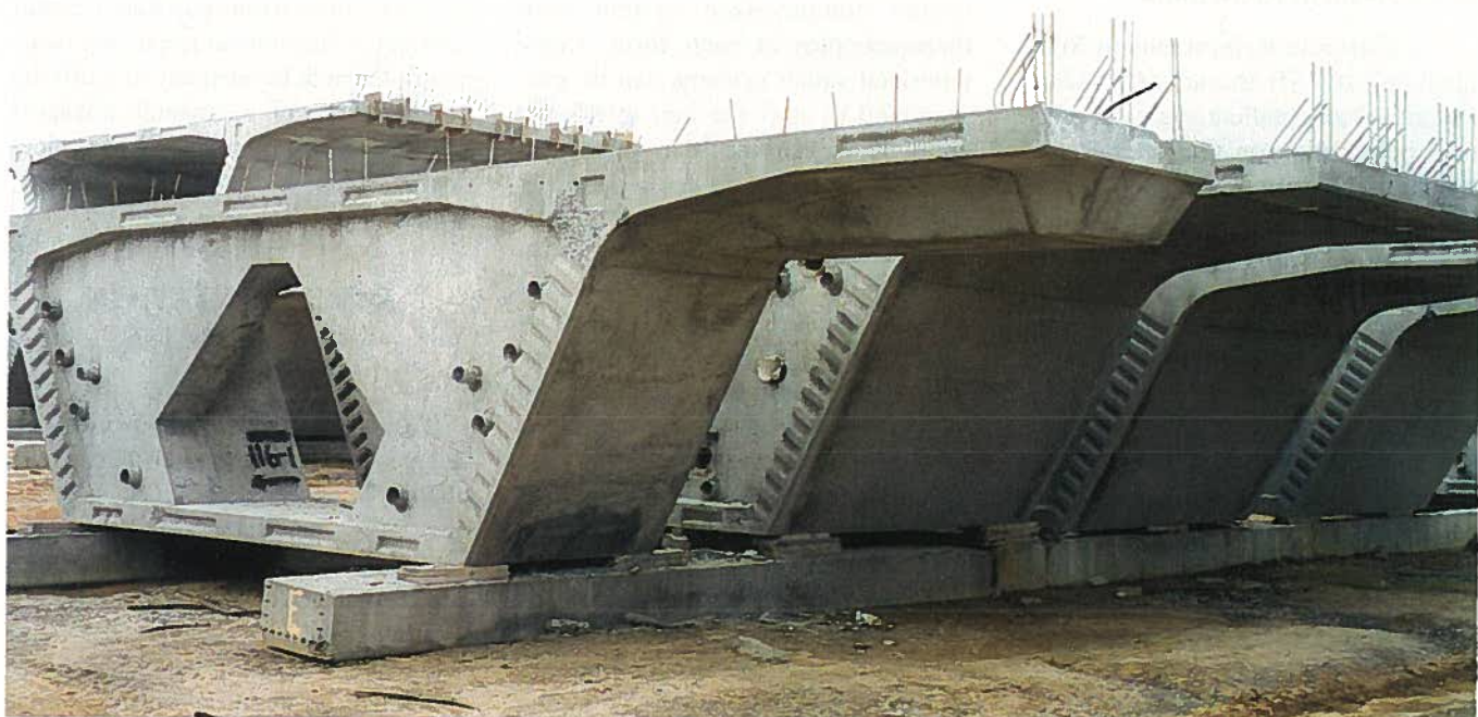
Fig. 2. Pier segments ready for shipment.
