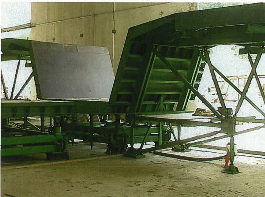
Fig. 4. Segmental casting machine setup before fixed bulkhead is installed.
