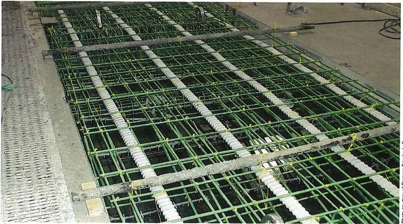
Fig. 8. Precise reinforcement and post-tensioning layout requirements produce excellent quality.
