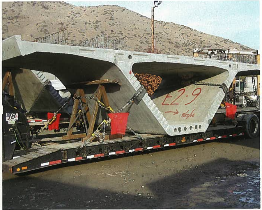
Fig. 9. Segment loaded on lowboy trailer ready for delivery.
