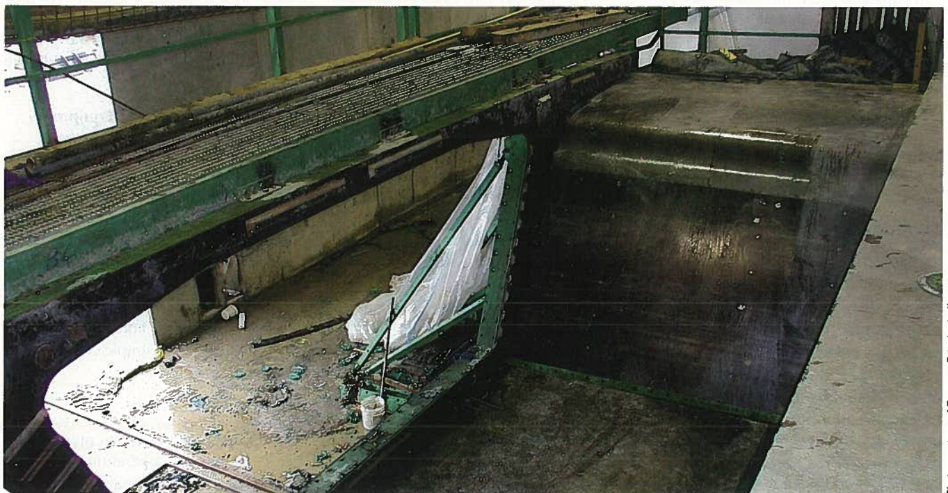
Fig. 7. Casting form prepped prior to placement of the reinforcing steel cage.
