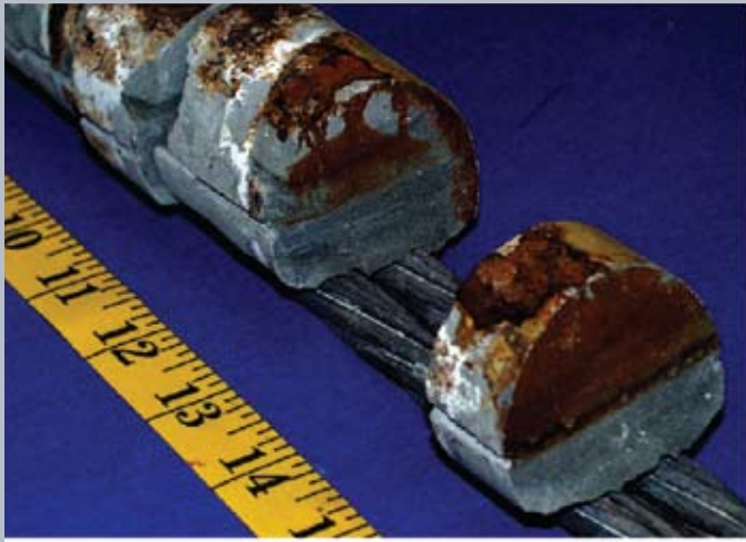
Figure 17. Pictured is the effect of grout cracking from the beam corrosion test series. Note: 1 in. = 25.4 mm.
