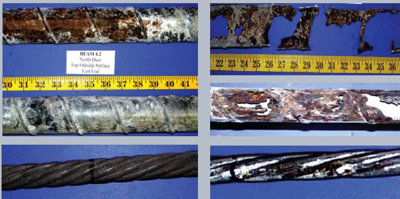
Figure 12. Pictured is corrosion in galvanized-steel duct in beams with different levels of post-tensioning from the beam corrosion test series. Note: 1 in. = 25.4 mm.
