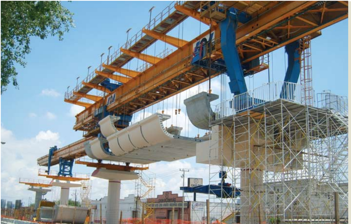
Figure 14. The spans were erected with two overhead gantries.
