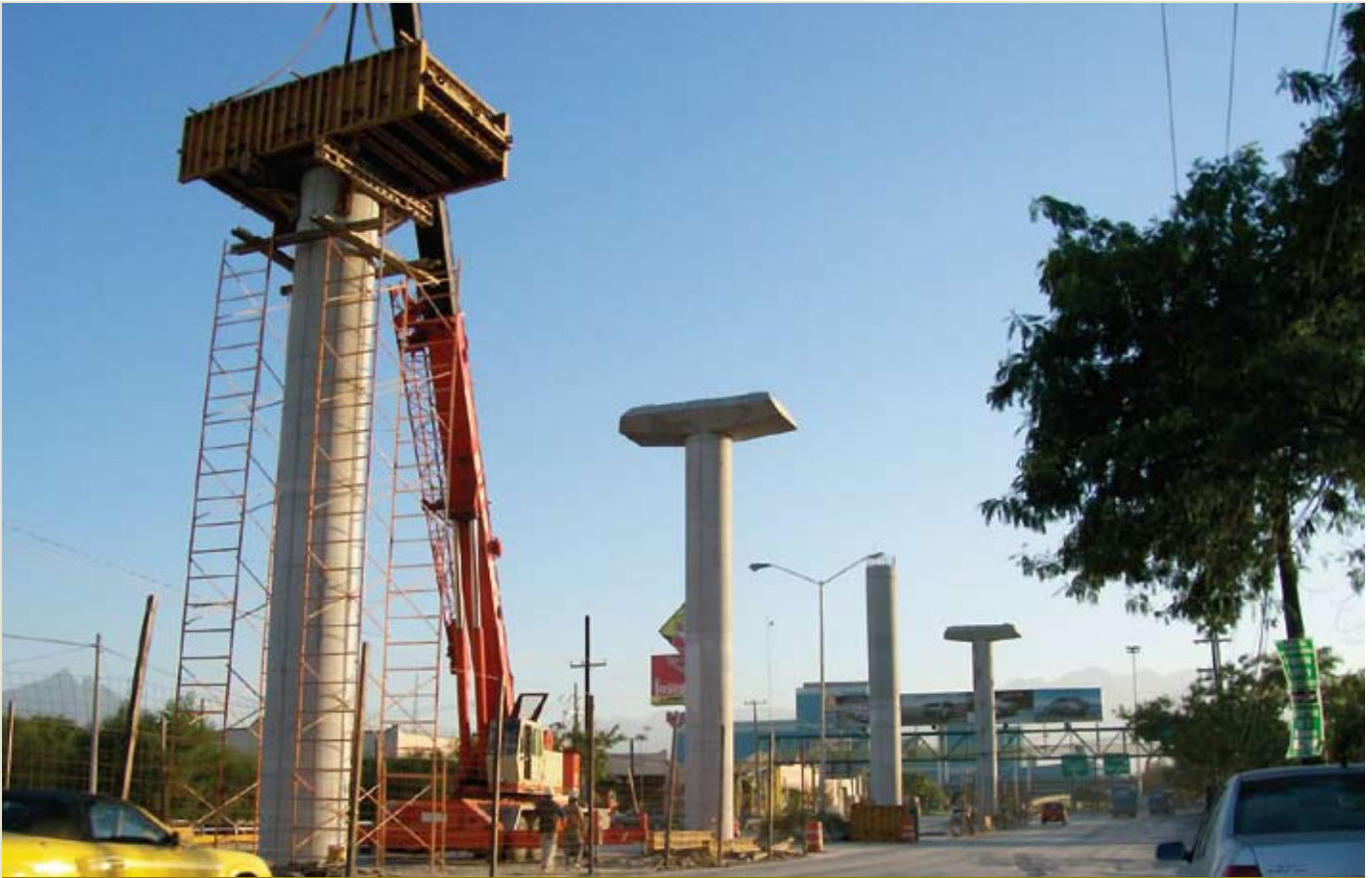
Figure 4. This photo shows the substructure of Metrorrey linea 2 during construction.
