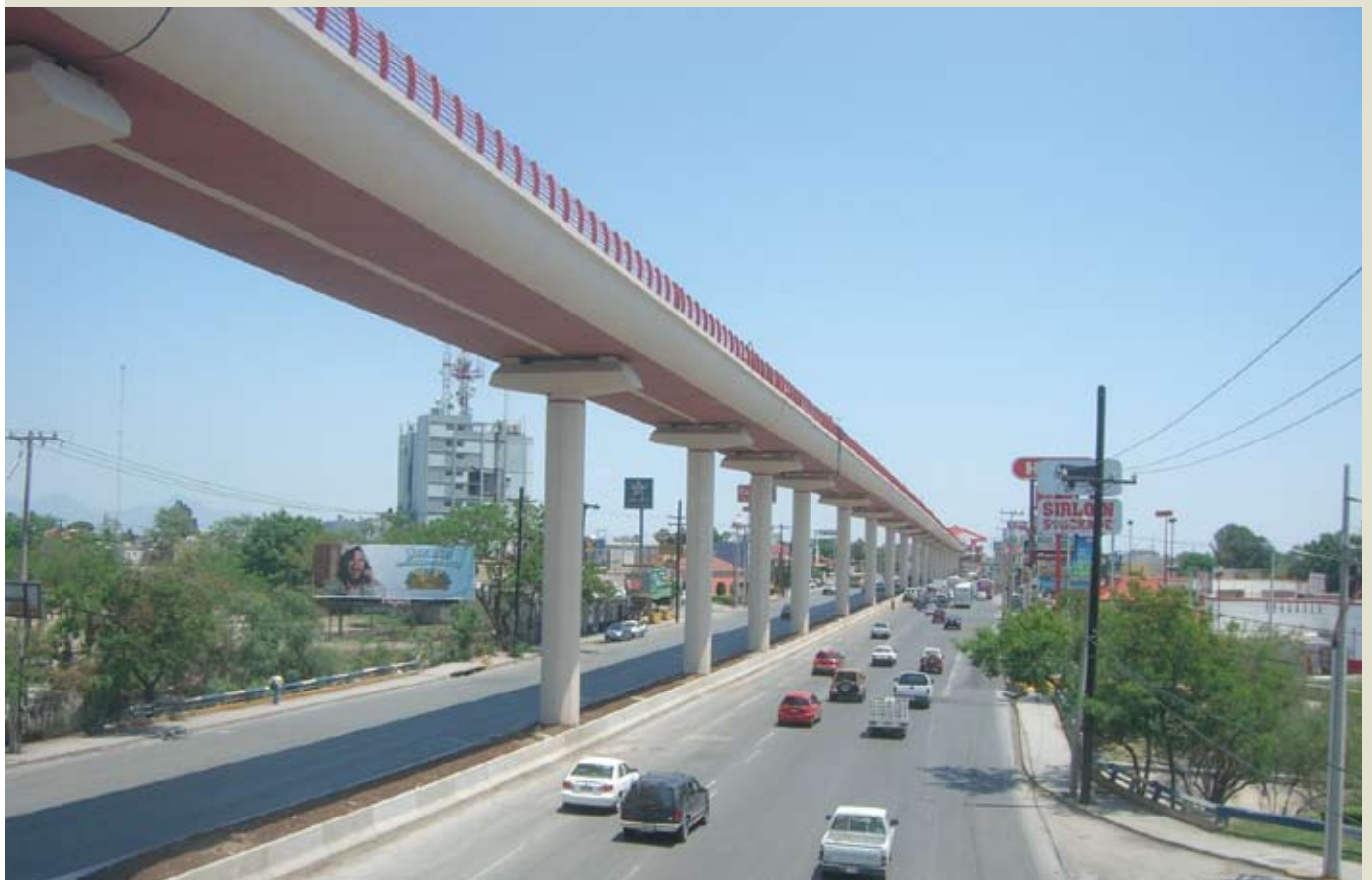
Figure 15. The completed spans here are on high-level piers.
