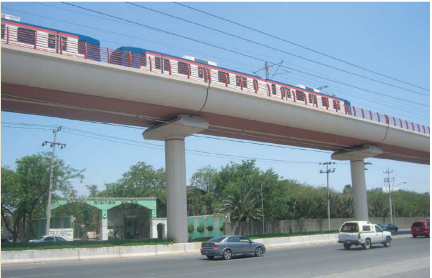
Figure 16. The completed spans here are on low-level piers.
