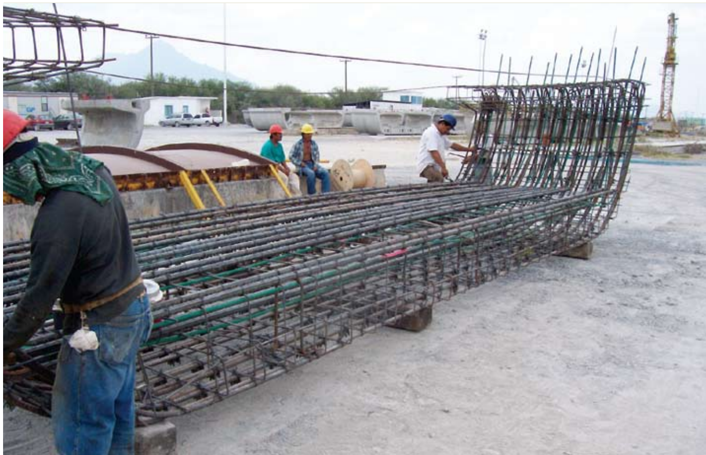
Figure 11. This photo shows the pier segment reinforcement.
