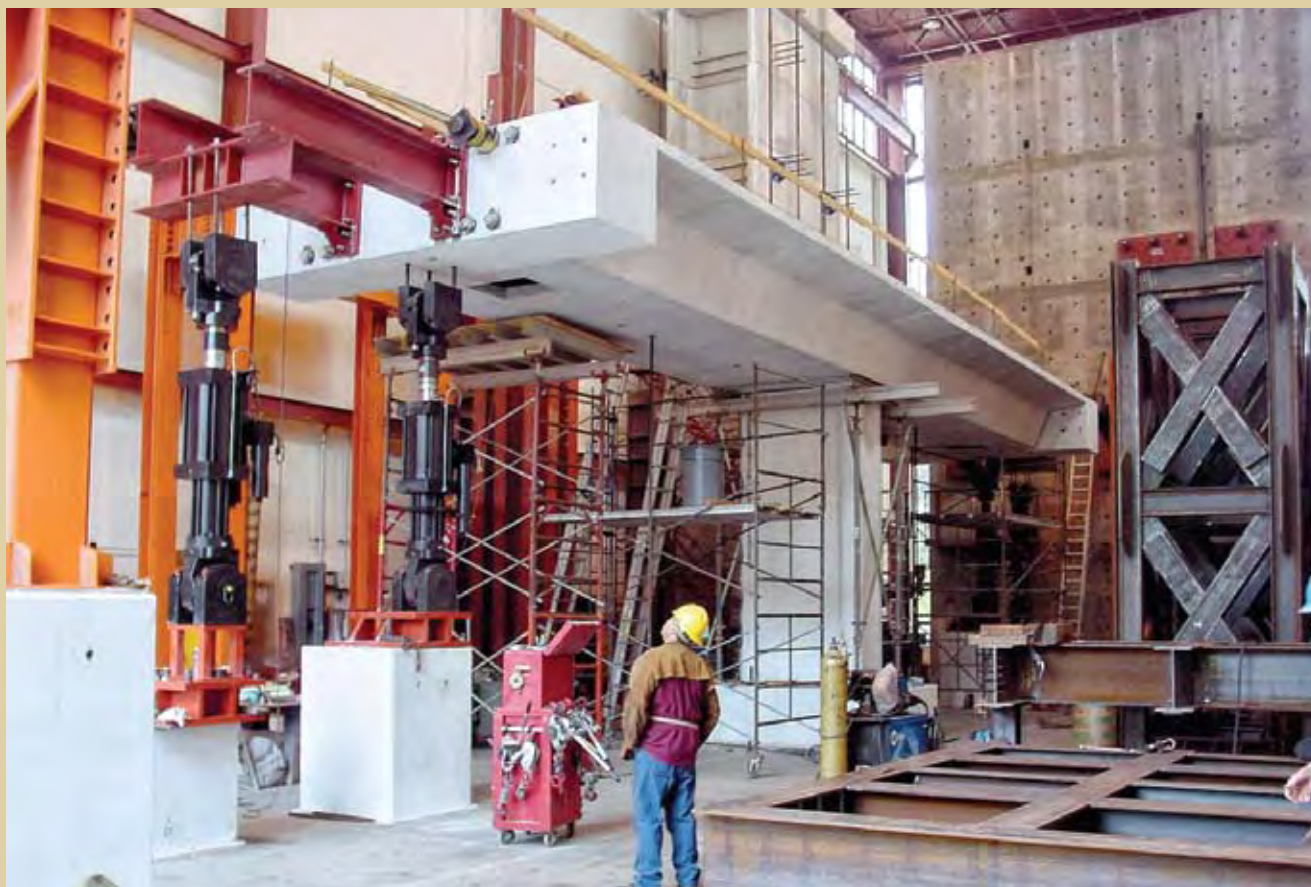
Figure 19. This drawing and photograph show the phase III test setup. Note: The drawing is not to scale. Source: Reprinted from Burnell, Megally, Restrepo, and Seible 2005. 1 in. = 25.4 mm; 1 ft = 0.305 m.
