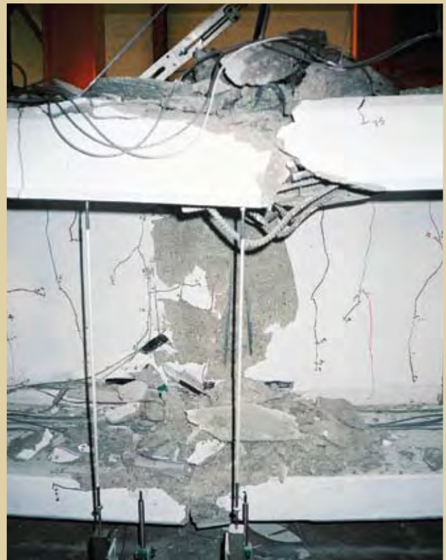
Test unit 100INTCIP brittle cast-in-place concrete deck buckling failure
