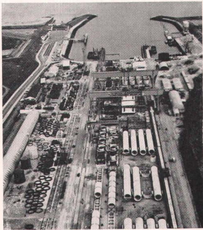
Fig. 2—Overall view of precasting facility for the Oosterschelde Bridge
