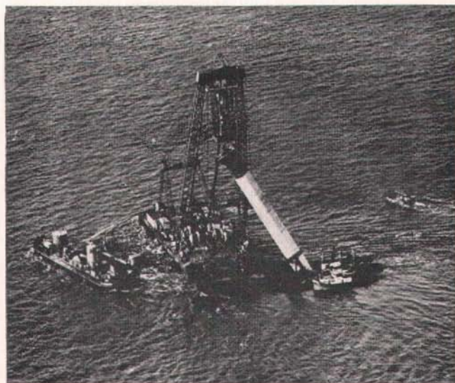
Fig. 5—Lifting a prestressed cylinder pile into position
