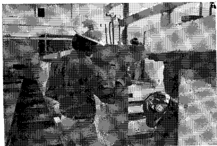
Fig. 4. Epoxy application.
