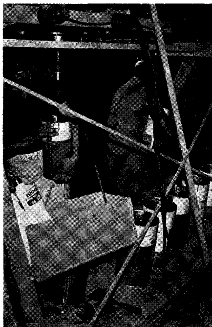
Fig. 7. Epoxy resin and hardener being readied for stirring (Rio-Niteroi Bridge, Brazil). In general, it is preferable to use a low-speed stirrer. On this job electric drill motors were mounted in line to mix six 11-lb batches of epoxy.
