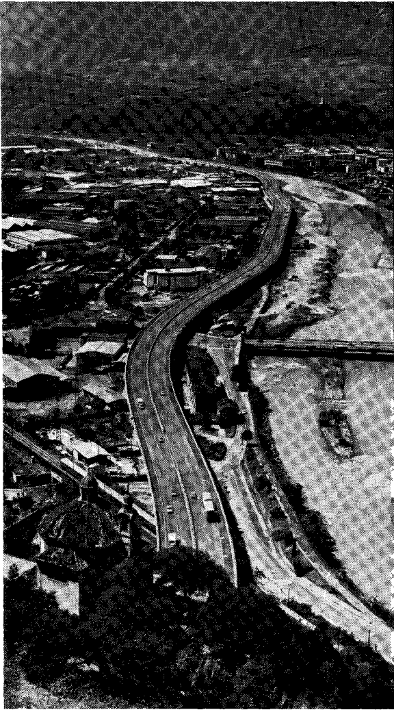
Fig. 1. Aerial view of elevated motorway.
