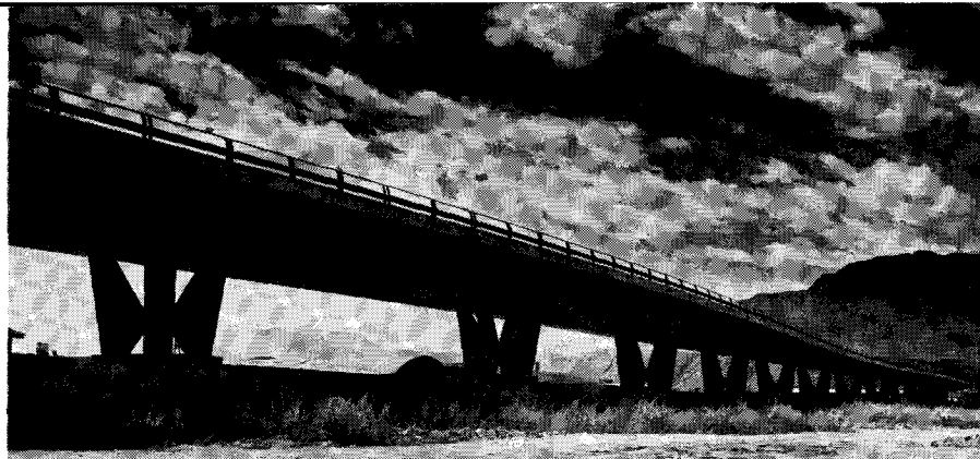
Fig. 23. Elevated motorway completed.
