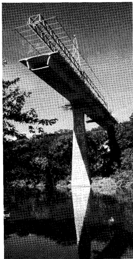
Fig. 17. This launching gantry is being used to erect the Kishwaukee River Bridge near Rockford, Illinois. This is the first such use of a launching gantry in the United States.
