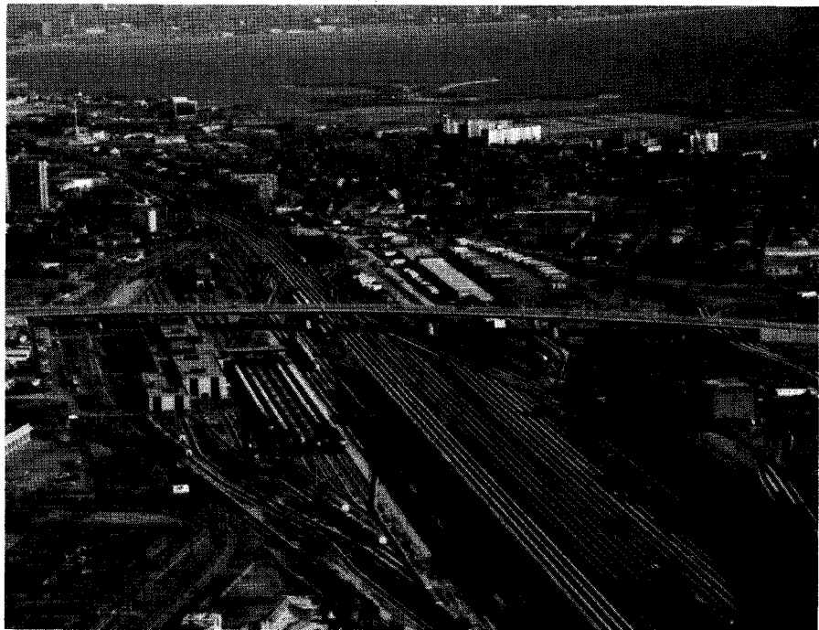
Fig. 18. Aerial view looking east at finished structure.
