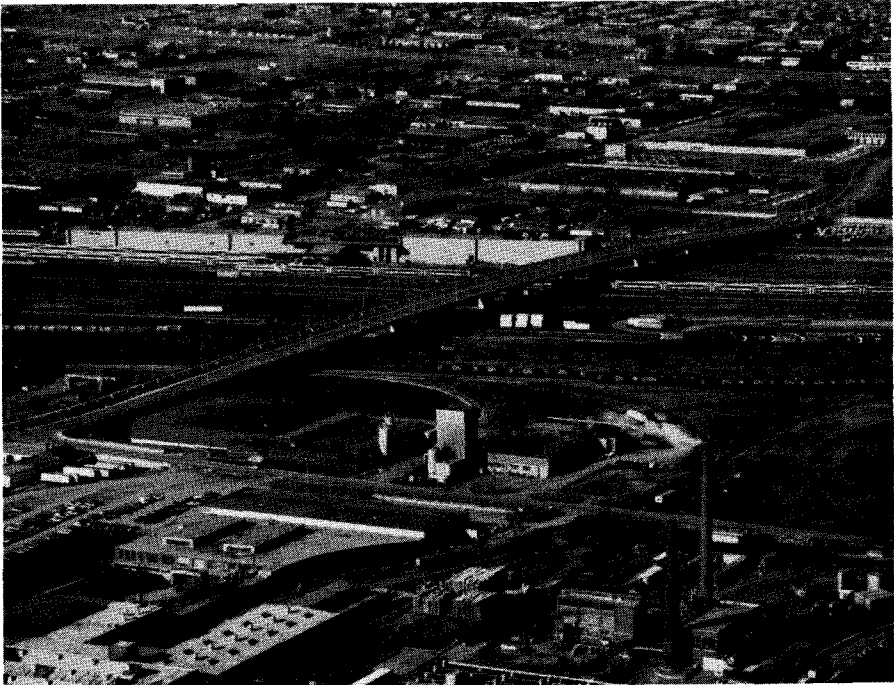
Fig. 19. Aerial view looking northwest at finished structure.
