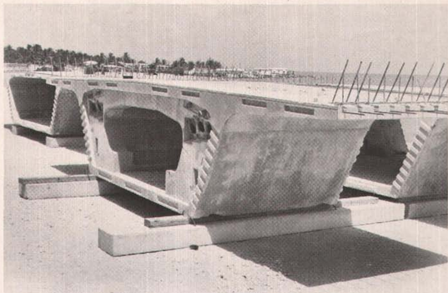
Fig. 17. Precast segments in storage yard waiting to be transported to erection site. Multiple shear keys and post-tensioning ducts can be seen. One purpose of the multiple shear keys is to obtain a more uniform transfer of shear stresses across match cast joints. Note that the joints between segments were dry (i.e., without epoxy).
