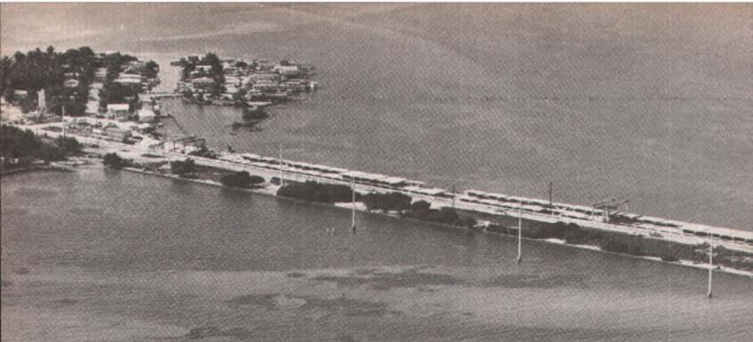
Fig. 10. Aerial view of casting yard with approximately 90 segments in storage.
