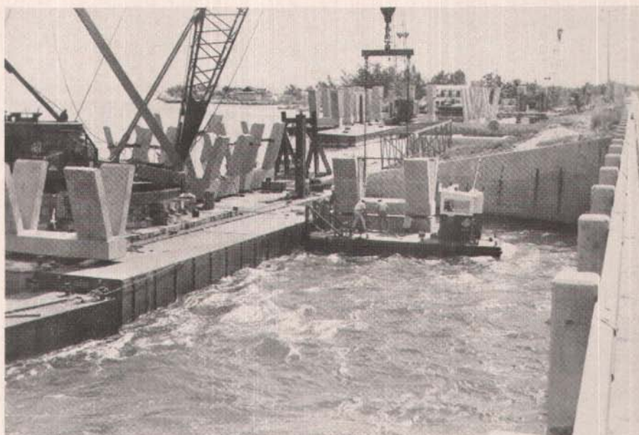
Fig. 13. First precast V-pier being placed on pile caps.
