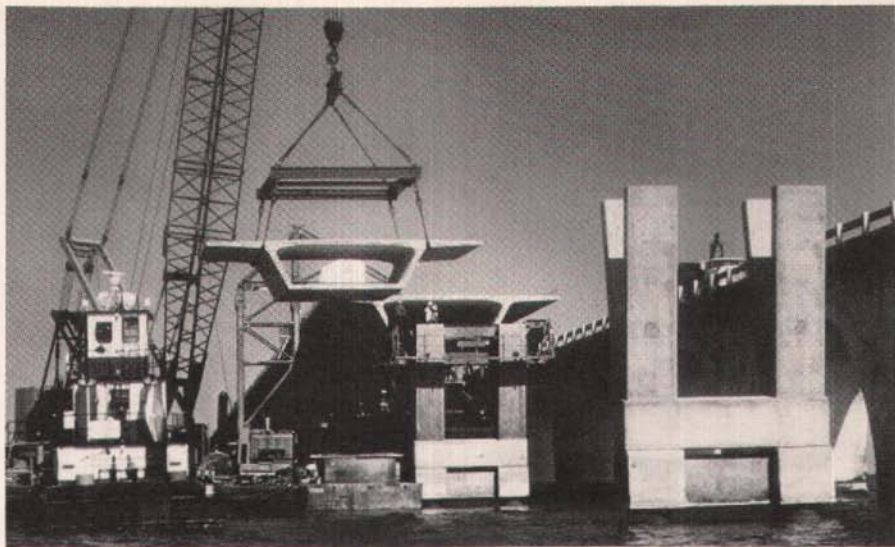
Placing precast segment with barge crane (Long Key Bridge).
