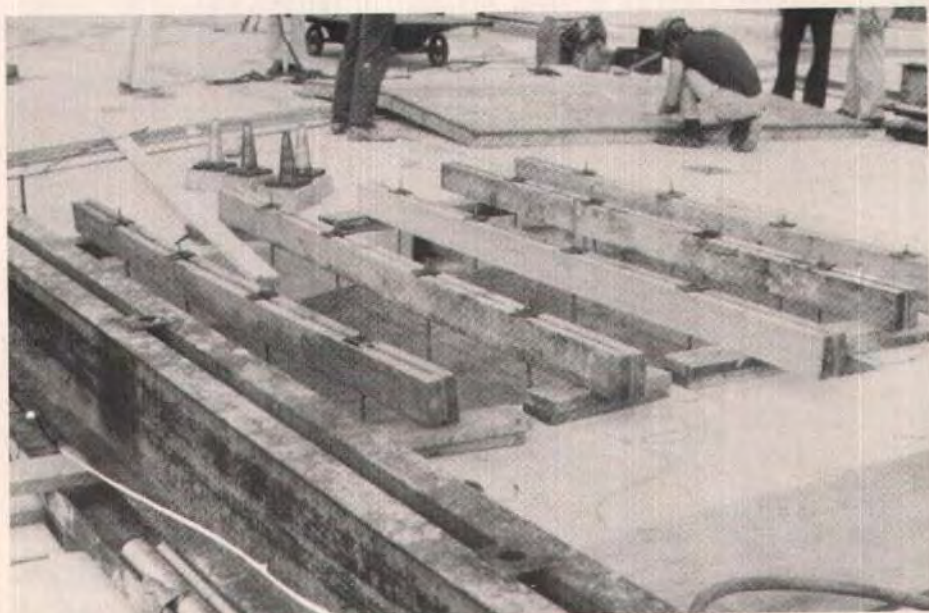
Fig. 26. The cast-in-place splices were formed and supported on the superstructure.
