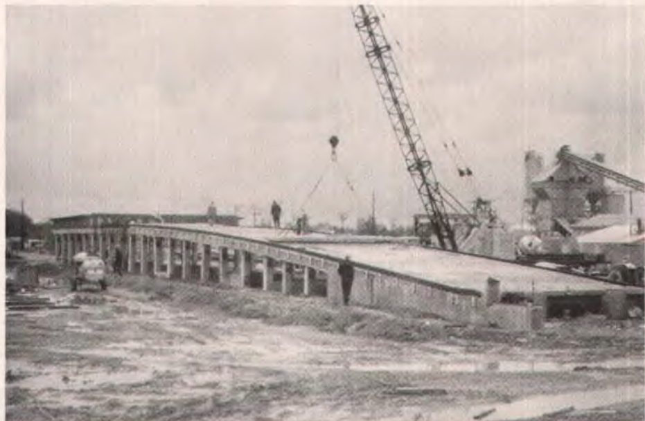
Fig. 8. Early construction of long-line casting bed in Henderson, Kentucky.
