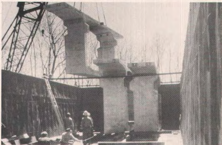
Fig. 17. The deeper segments were loaded on barges.
