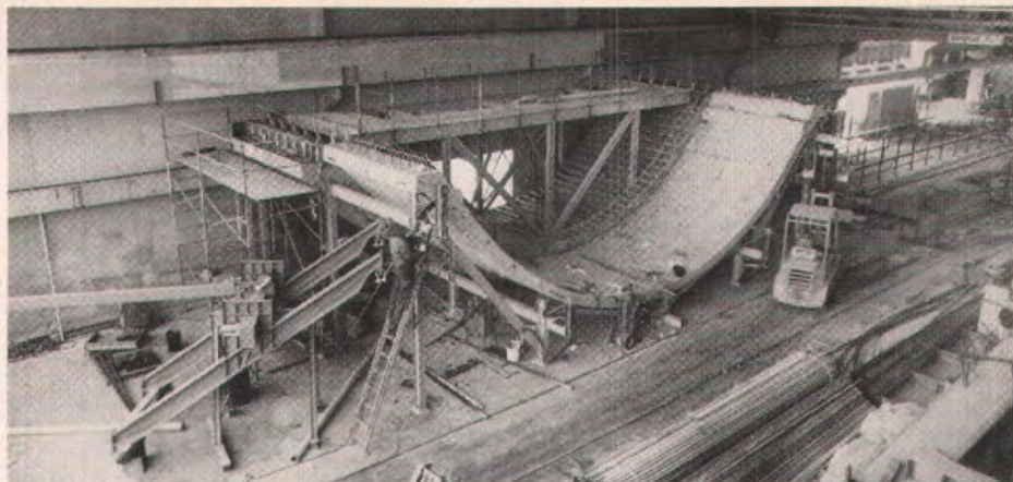
Fig. 10. Match-casting, precast concrete bottom shell segments.
