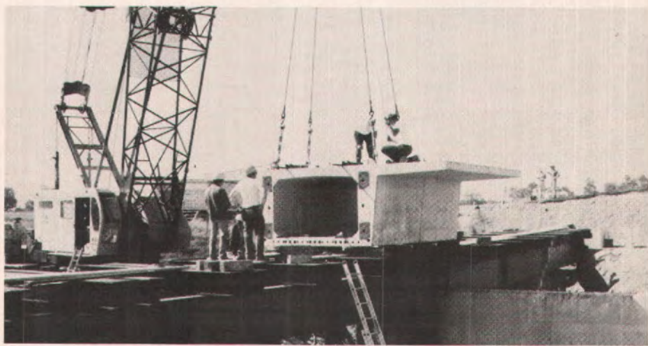
Fig. 16(b). Span-by-span technique using falsework at Pennsylvania Transportation Research Facility.
