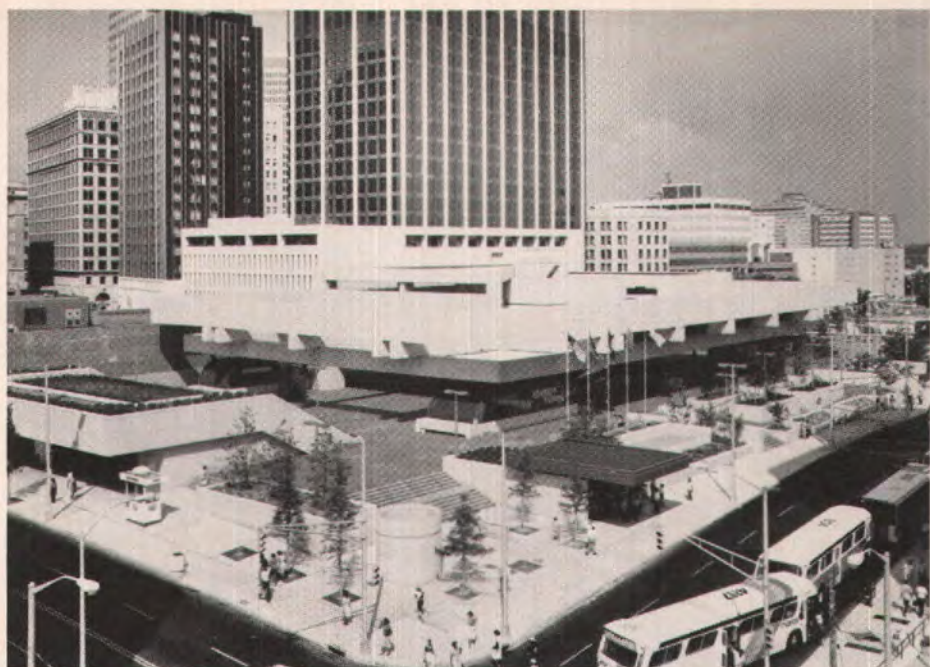
Fig. 13. Five Points Station, Atlanta Rapid Transit System, Atlanta, Georgia.
