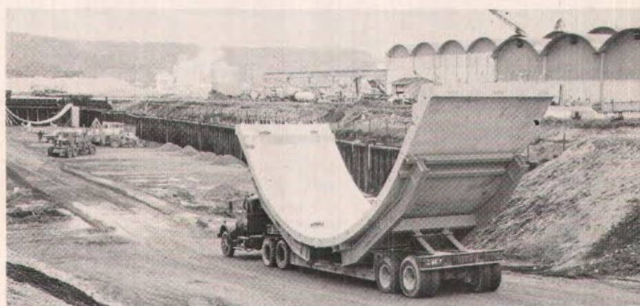
Fig. 11. Graving dock and delivery of 40-ton bottom hull segment.
