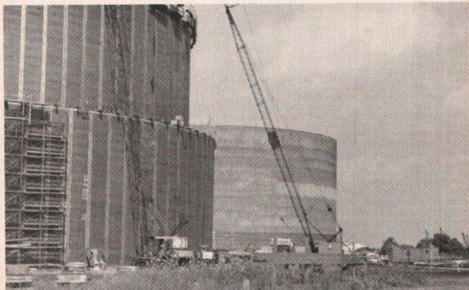
Fig. 4d. Overall view of LNG tanks during construction.
