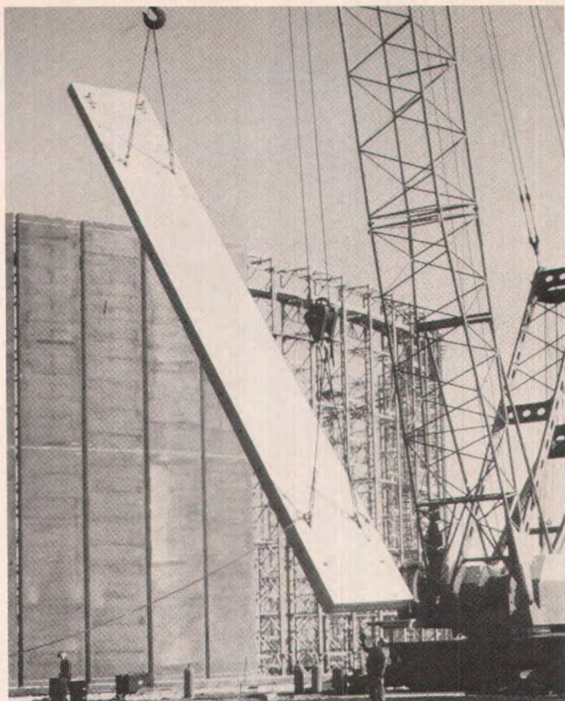
Fig. 3. Erection of precast panel for liquid natural gas storage tank.
