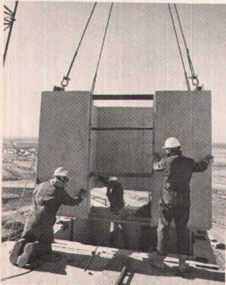
Fig. 1(c). Setting of box segments.
