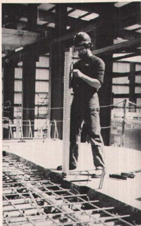
Fig. 10. Positioning the old segment (Zilwaukee Bridge, Michigan).
