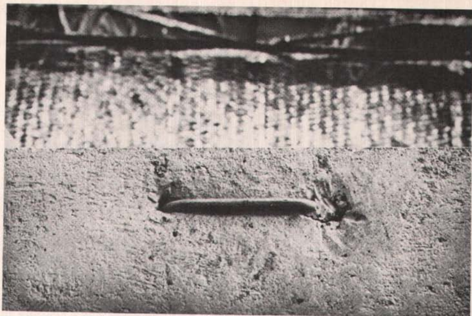
Fig. 8. Match-cast segment showing centerline marker.
