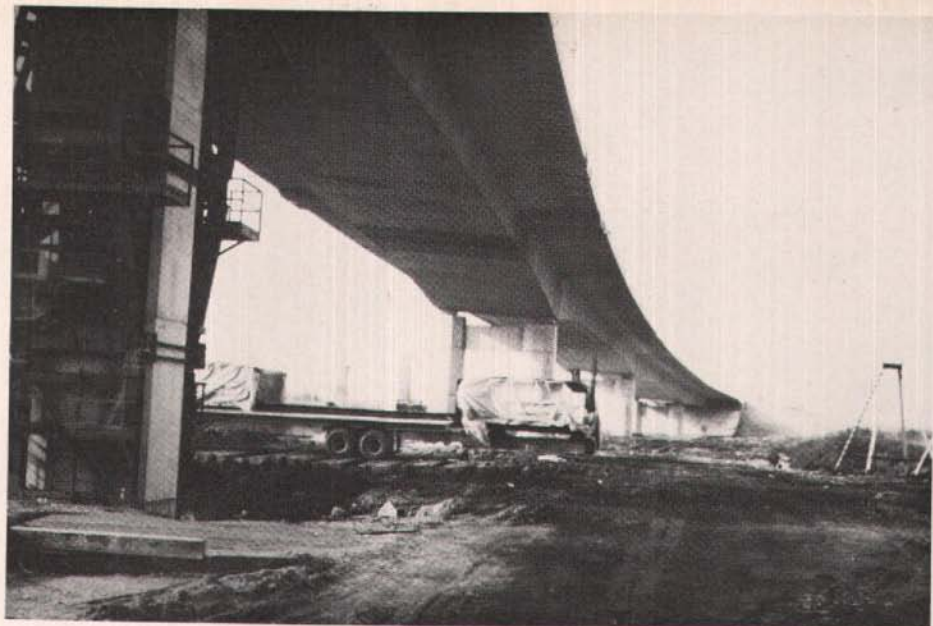
Fig. 17. Horizontal curve (Zilwaukee Bridge, Michigan).
