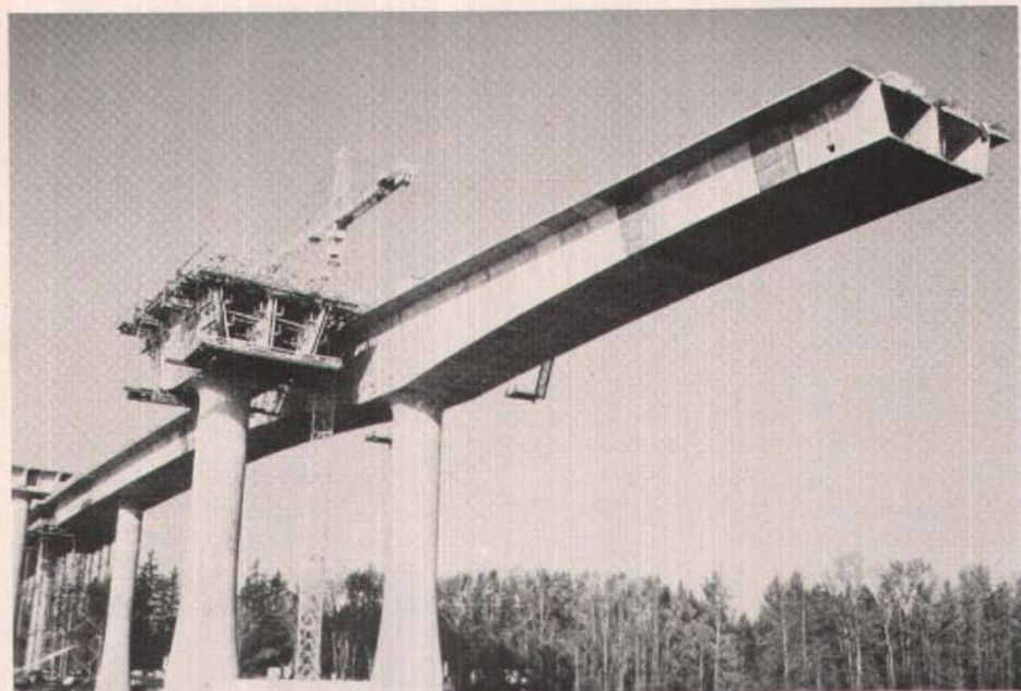
Fig. 1. Main span of I-205 Columbia River Bridge.
