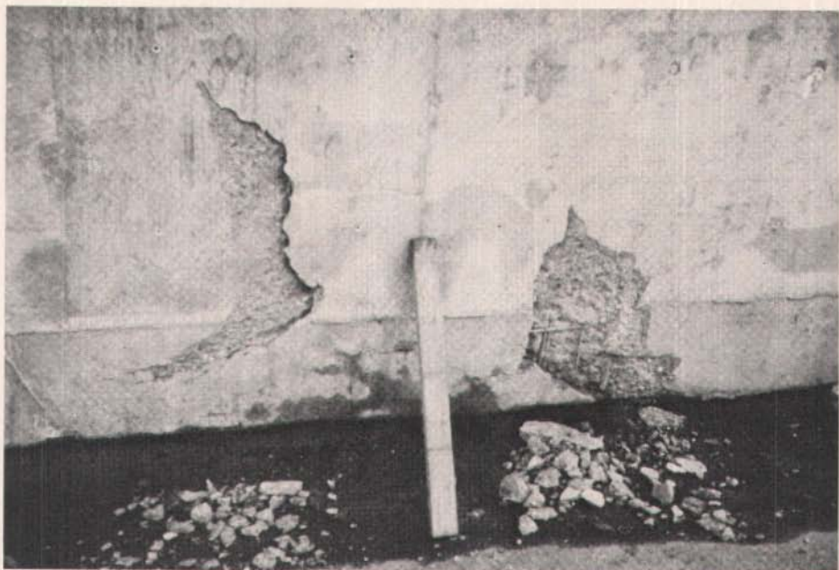
Fig. 2. Water freezing in ducts.
