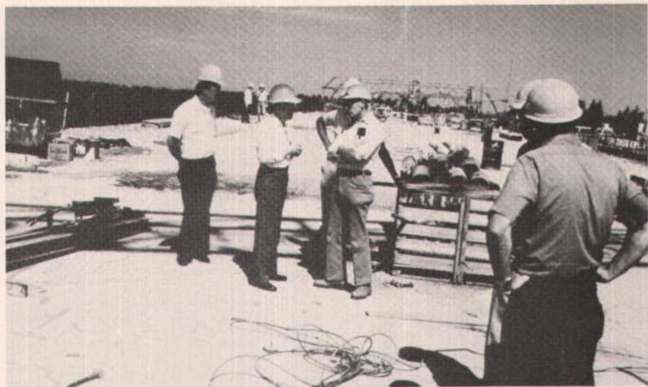
Fig. 7. Inspecting the laminar cracks in deck.
