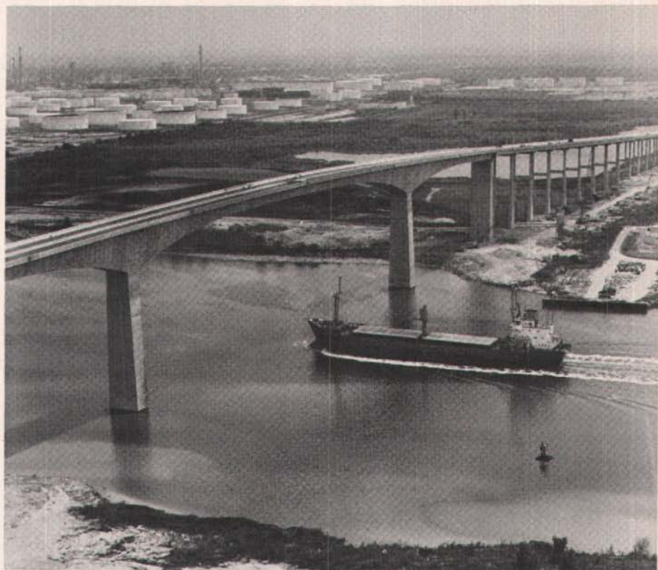
Fig. 22. Houston Ship Channel Bridge in use.
