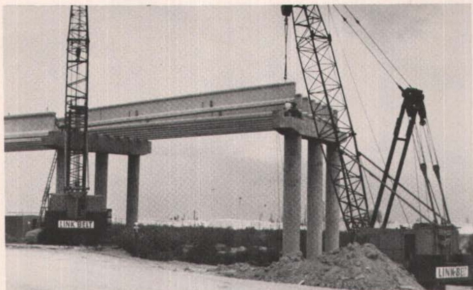
Fig. 8. Placing AASHTO type beams on land approaches.
