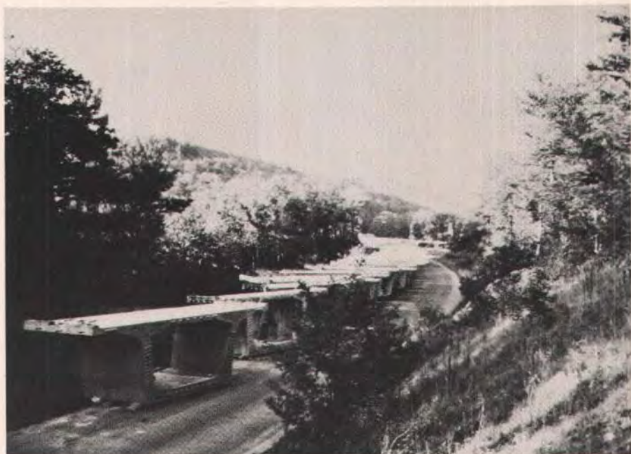
Fig. 5. Typical yard storage along road leading to bridge site.
