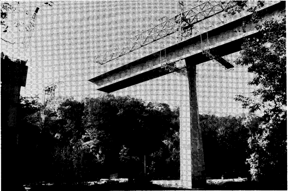
Fig. 11. Kishwaukee River Bridges, Winnebago County, Illinois, during construction.
