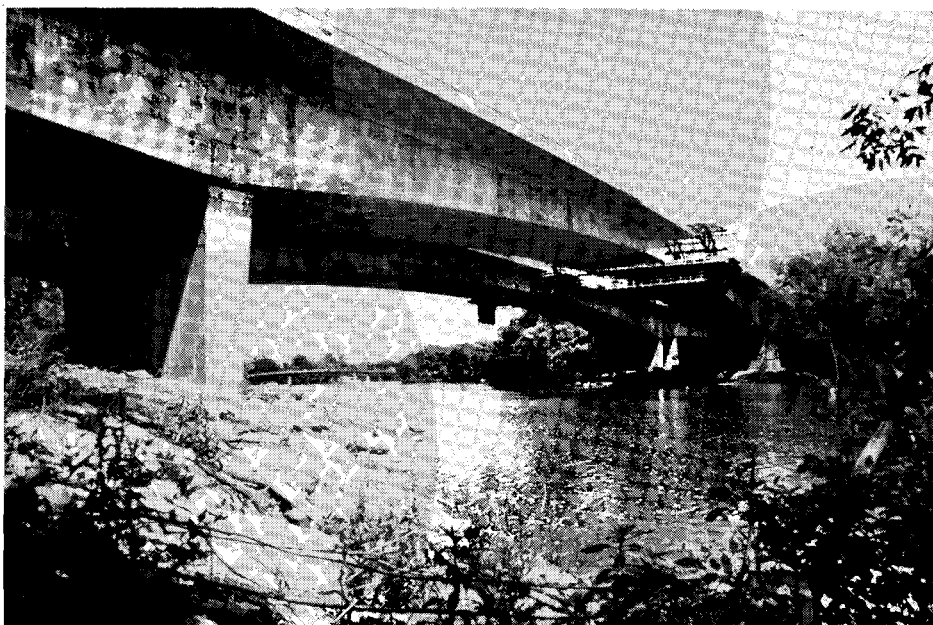
Fig. 13. Genessee River Bridge, Rochester, New York.
