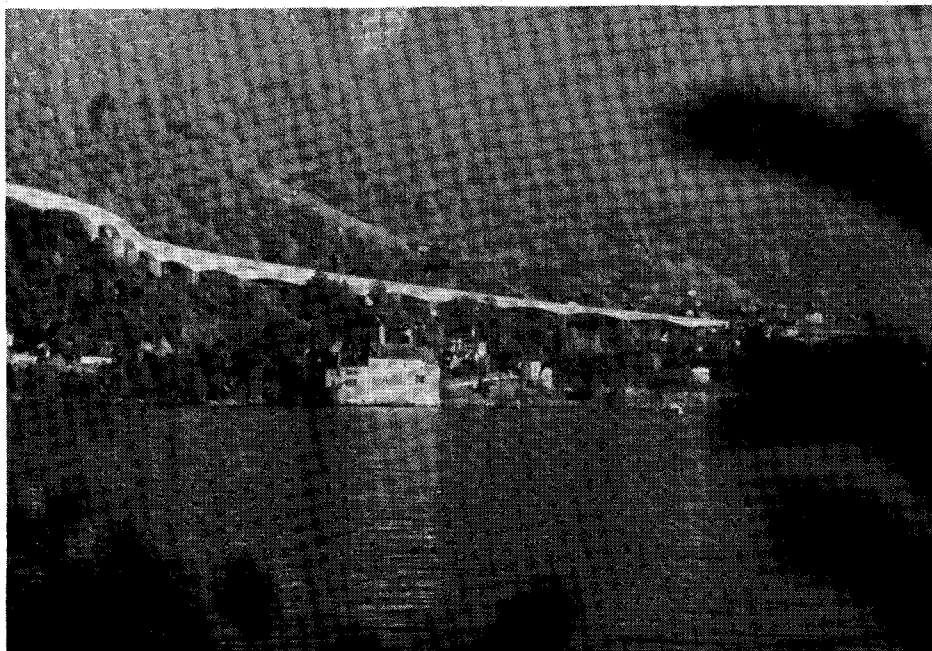
Fig. 19. Chillon Viaduct, Switzerland.
