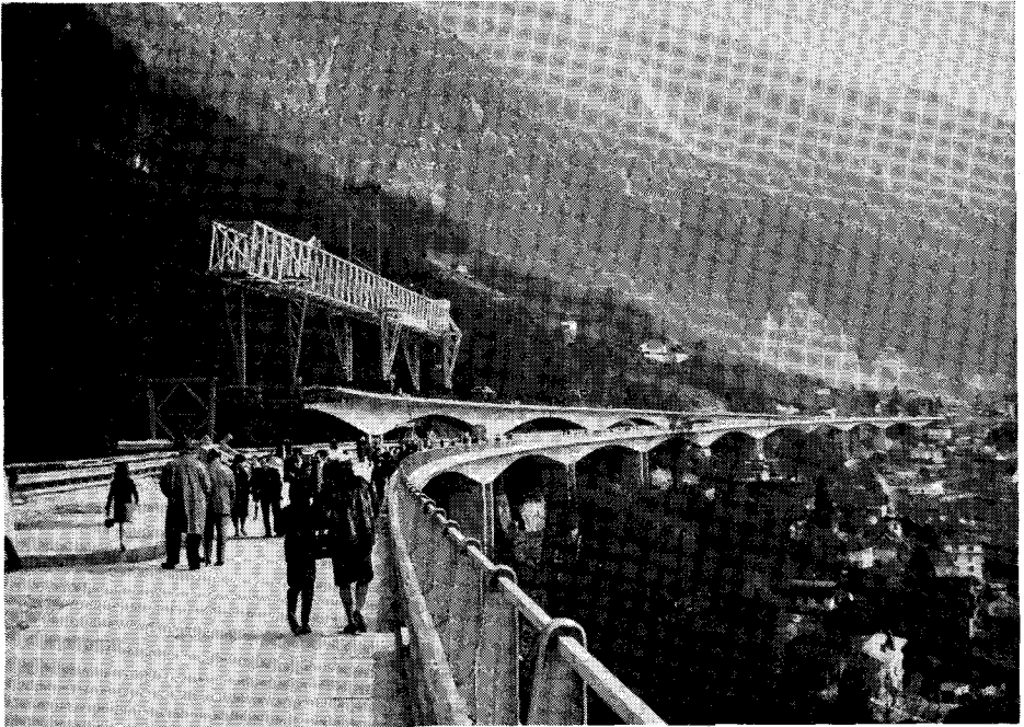
Fig. 20. Chillon Viaduct, Switzerland.
