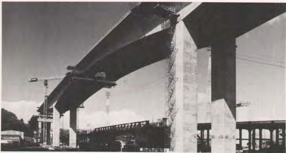
Fig. 12. West Seattle Bridge, nearing completion.
