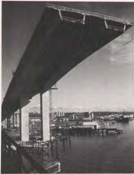
Fig. 11. West Seattle Bridge, halfway through construction.
