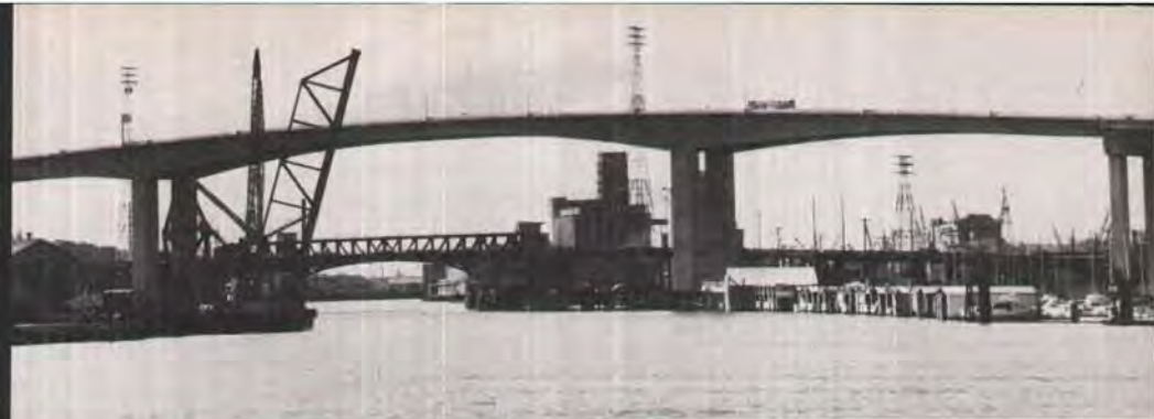
Fig. 13. West Seattle Bridge, completed and in-service.
