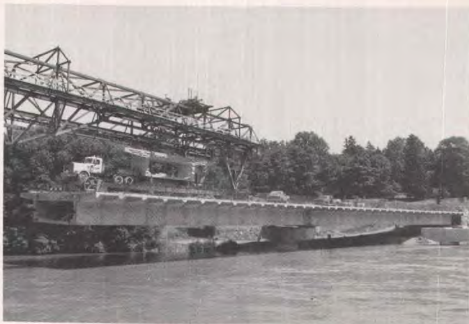
Fig. 11. Delivering segment on completed cantilever for erection by launching truss.
