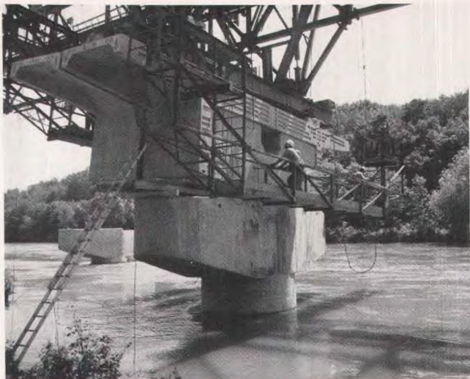
Fig. 10. Typical pier segment with cast-in-place diaphragm and erection of adjacent segment.
