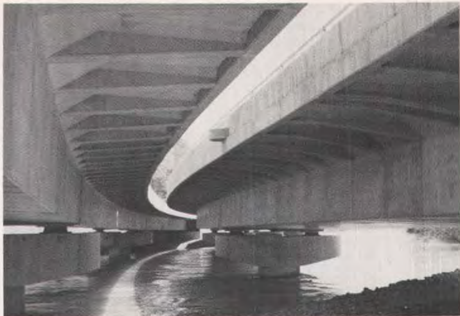
Fig. 12. Underside view of completed bridges showing the transverse ribs.
