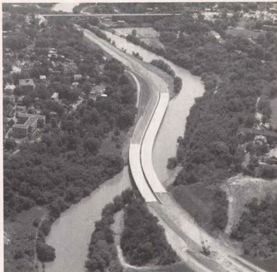
Fig. 1. Aerial view of the completed bridges.
