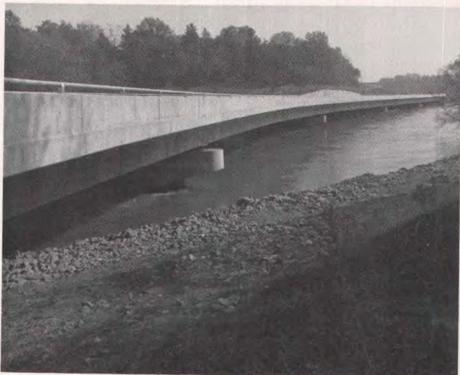
Fig. 13. View of completed bridge.
