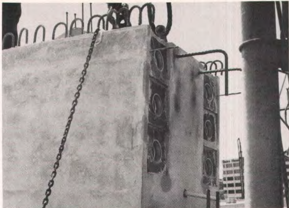
Fig. 9. End view of one of the segments. Note the three ducts and base plates in each side wall.
