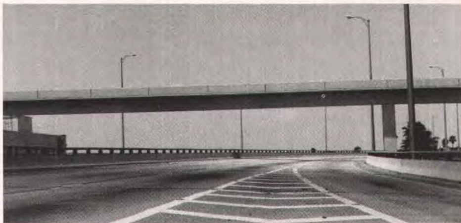
Fig. 1. Segmental span of the Harbour Island People Mover which links the mainland of downtown Tampa with Harbour Island, a billion dollar commercial development.
