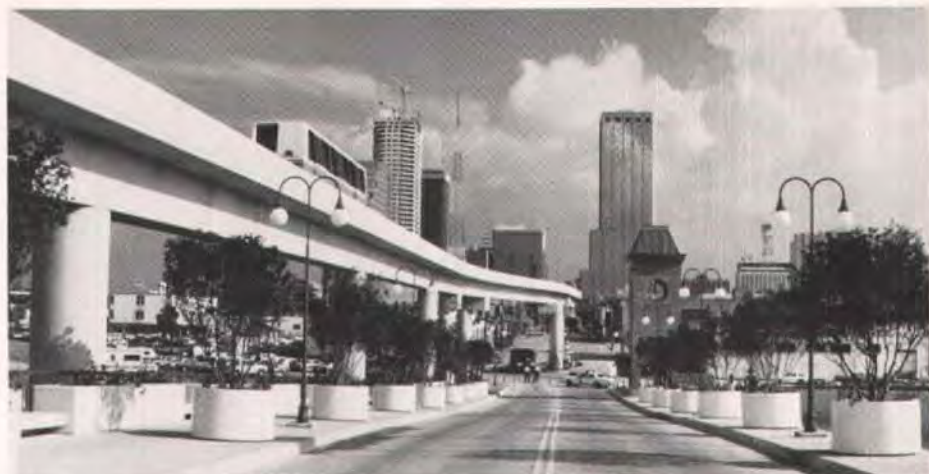
Fig. 11. Finished view of Harbour Island People Mover which is now fully operational.
