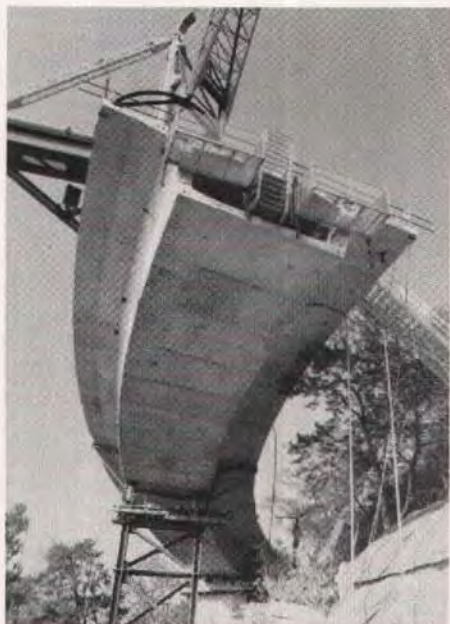
Fig. 15. Erection progress (May 20, 1982).
