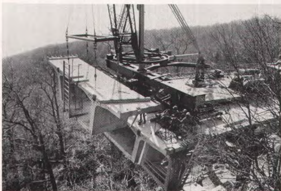
Fig. 13. Then the segment was lowered vertically.
