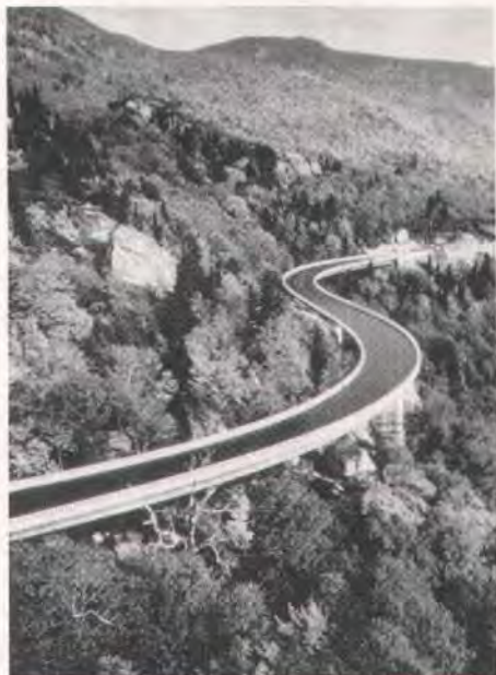
Fig. 16. Linn Cove Viaduct winding through the Blue Ridge Mountains.
