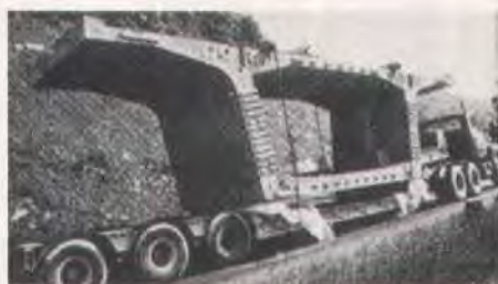
Fig. 10. 50 ton (45 t) segments had to be backed for distances exceeding 1 mile (1.6 km) in many instances because there was insufficient room to turn this rig around.
