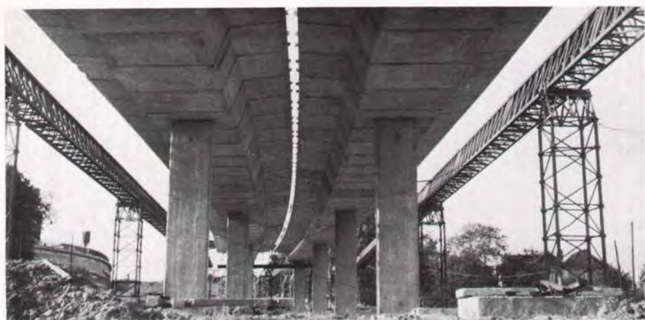
Fig. 18. Construction of DS-W type bridge in Brno-Reckovice, Czechoslovakia.
