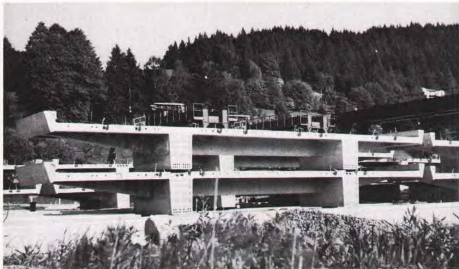
Fig. 24. Segments of a DS-T type bridge.
