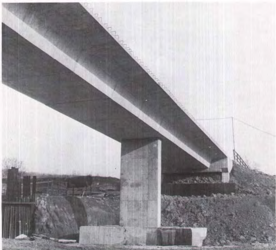
Fig. 7. Continuous box girder bridge.
