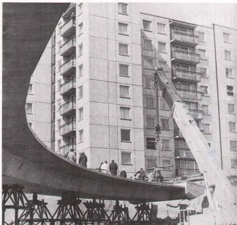
Fig. 14. Erection of the end cross beam.
