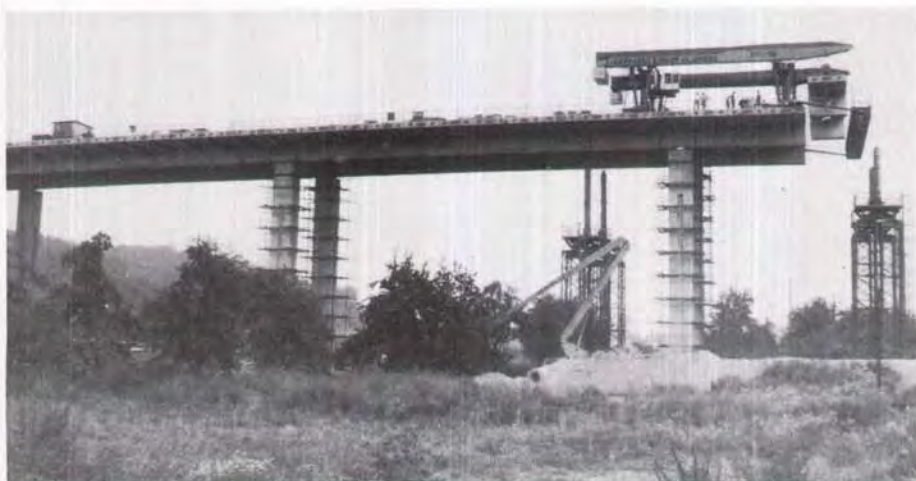
Fig. 32. Erection of bridge segments across the Rokytká River in Prague.
