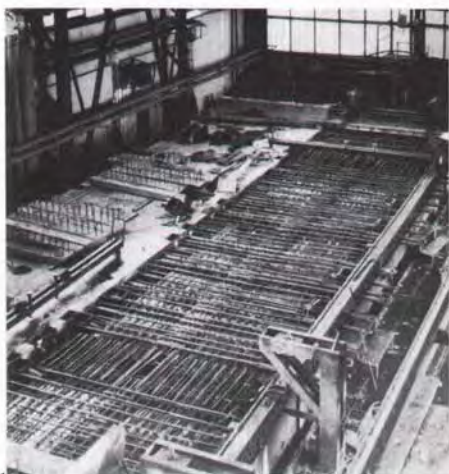
Fig. 26. Forms for DS-T type segments.
