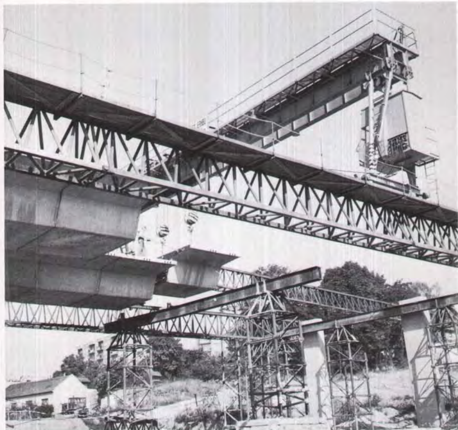
Fig. 21. Erection of DS-W segment by a portal crane.
