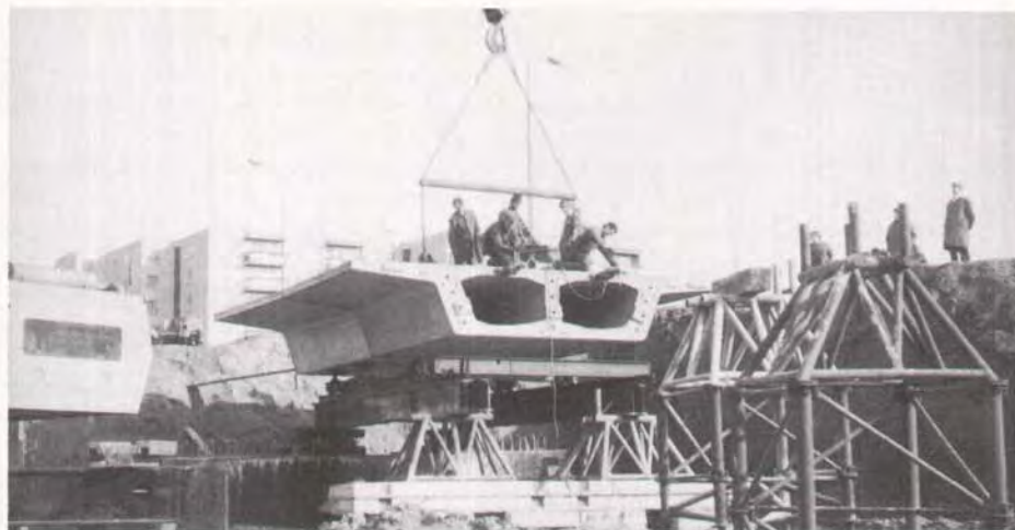
Fig. 13. Post-tensioning of the first two segments.
