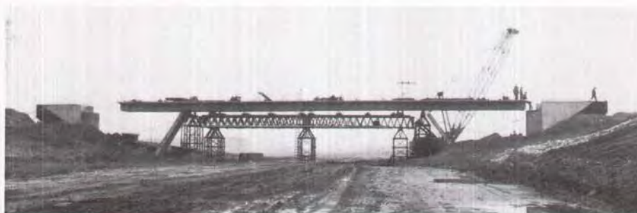
Fig. 4. Erection of side spans of overpass bridge.
