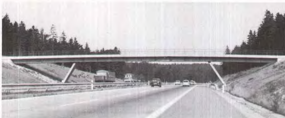
Fig. 3. Overpass bridge across the Highway Prague-Brno.
