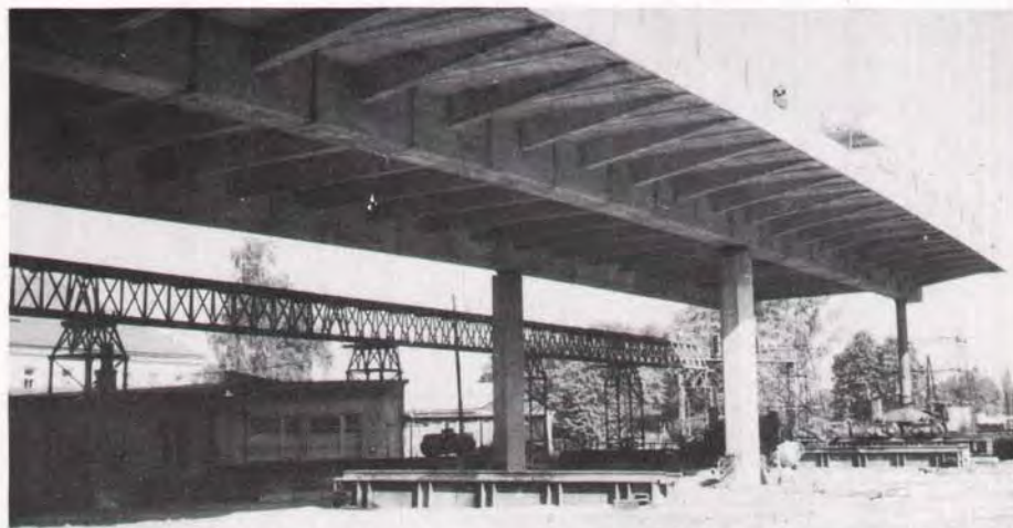
Fig. 30. Temporary support of DS-T type bridge at Valasske Mezirici.
