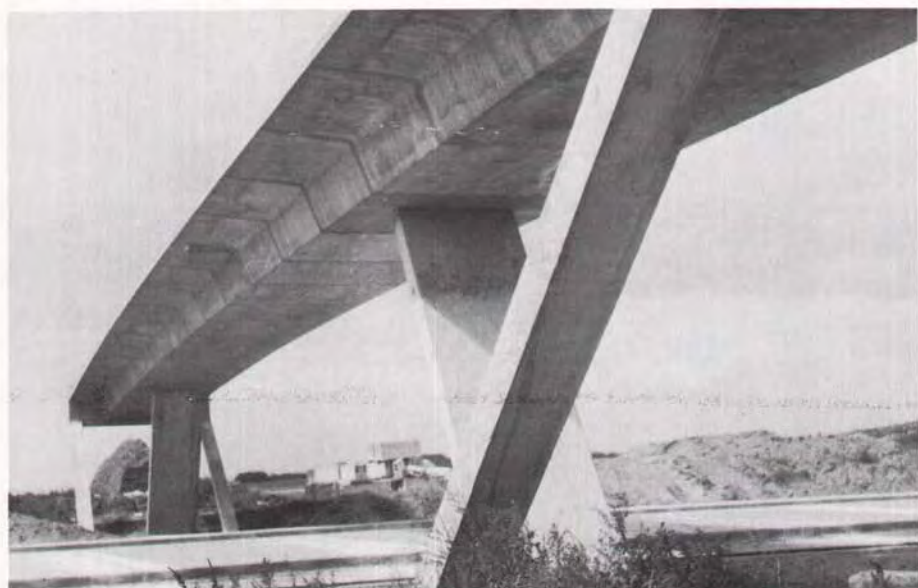
Fig. 8. Slant leg portal frame.
