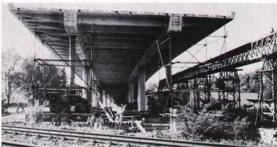
Fig. 29. DS-T type bridge at Valasske Mezirici during construction.
