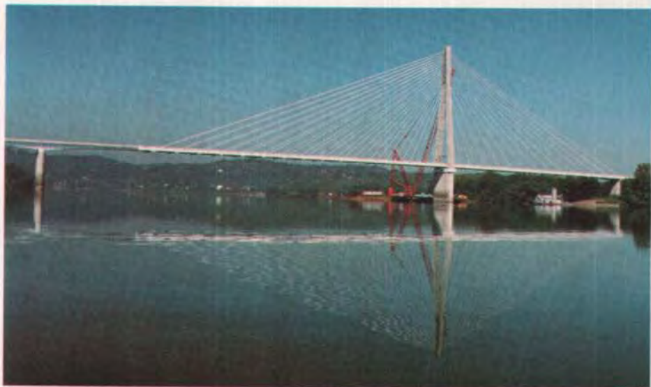
Fig. 9. Nearly completed East Huntington Bridge.
