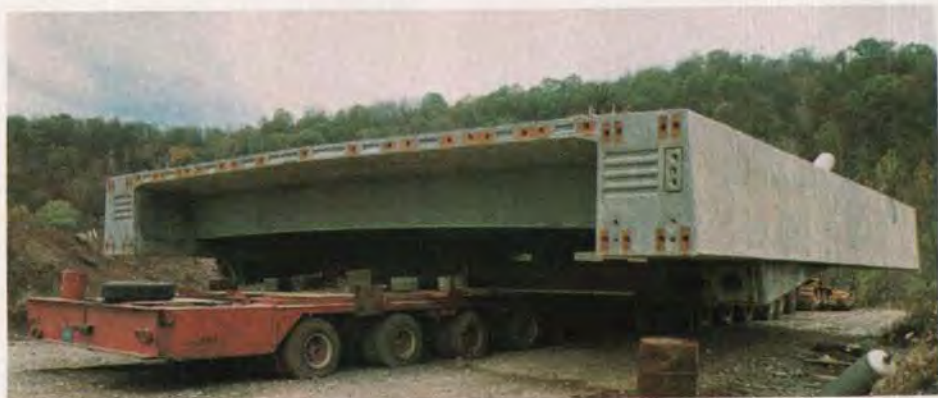
Fig. 3. A 250 ton (227 t) precast girder segment being transported to project site.
