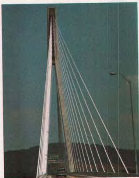
Fig. 11. Roadway view of the East Huntington Bridge.
