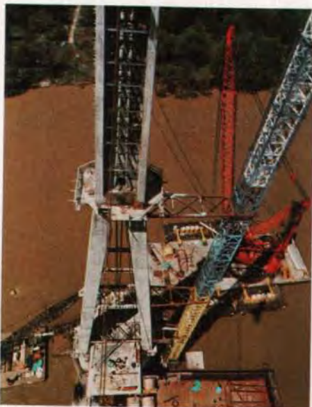
Fig. 5. Aerial view of tower.
