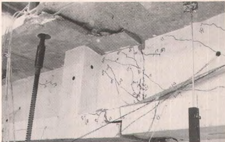
Fig. 13. Joint 7-8 of the Modified Unbonded Tendon Girder after testing.
