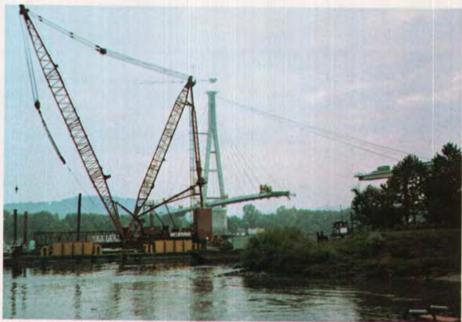
Fig. 7. Barge crane for segment erection.
