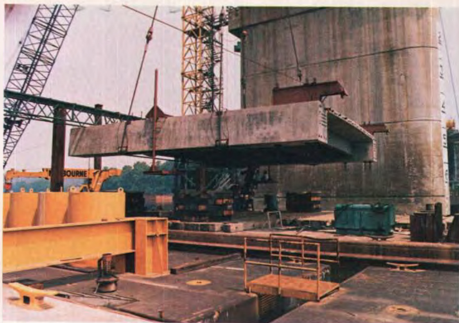
Fig. 11 (top and bottom). Views of segment erection.
