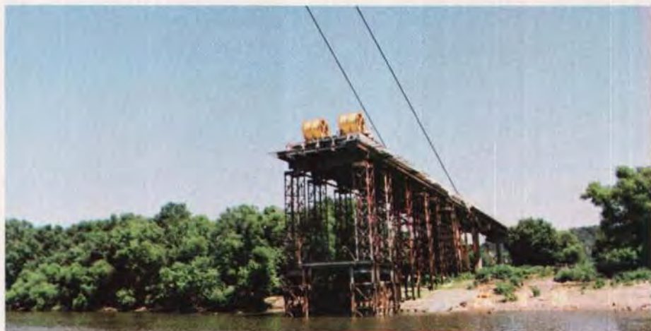
Fig. 10. Falsework support for end segments.
