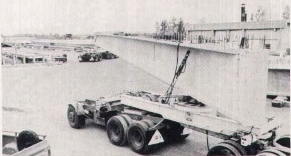
Fig. 6c. Transportation of long span beam.
