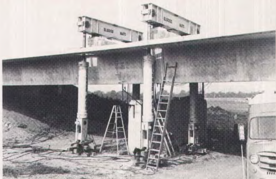
Fig. 8. The loading frame of the bridge.
