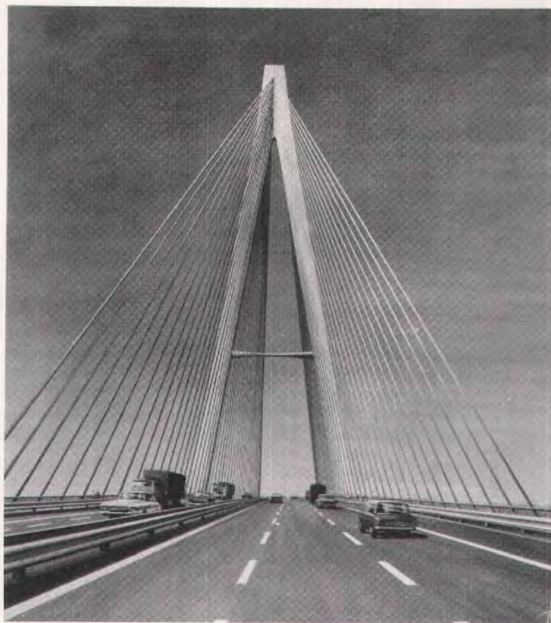
Fig. 20. View of A-shaped tower as motorist approaches bridge. There is an inherent feeling of comfort and safety.
