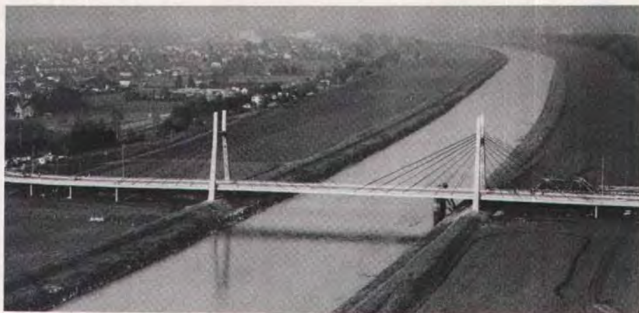
Fig. 25. Bridge across the Rhine at Diepoldsau, West Germany. Span = 97 m (318 ft).
