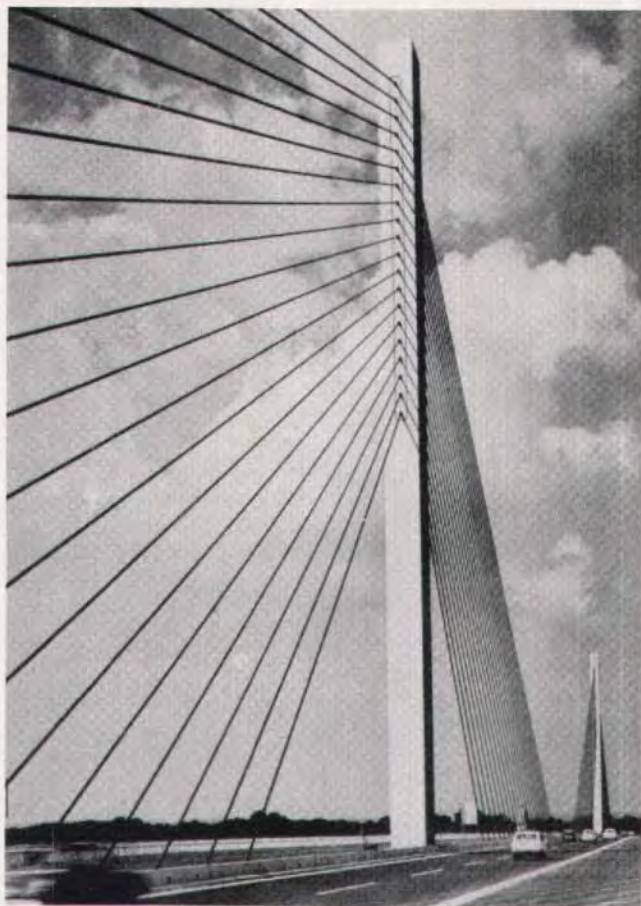
Fig. 21. Tower in median of Rhine Bridge in Bonn-Nord, West Germany.
