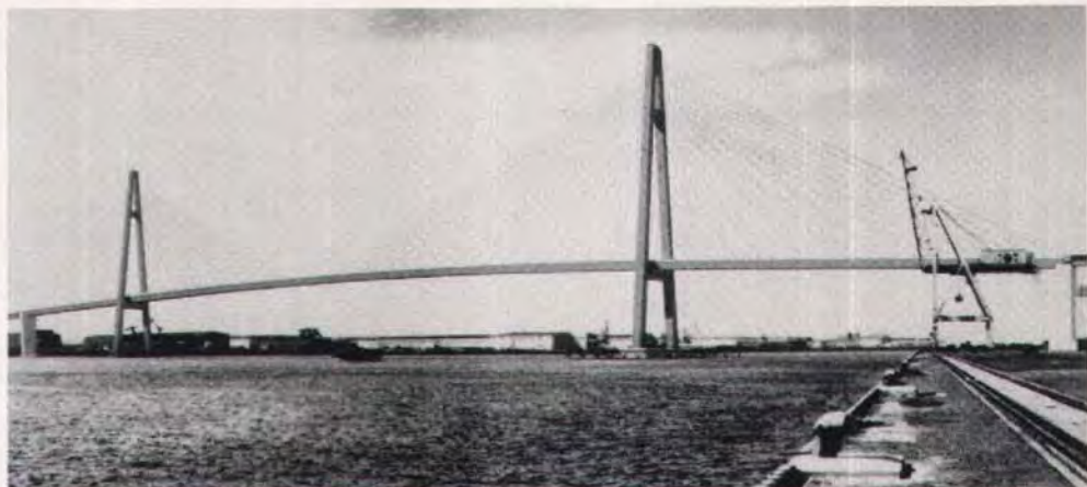
Fig. 3. Nagoya Harbour Bridge, Japan.
