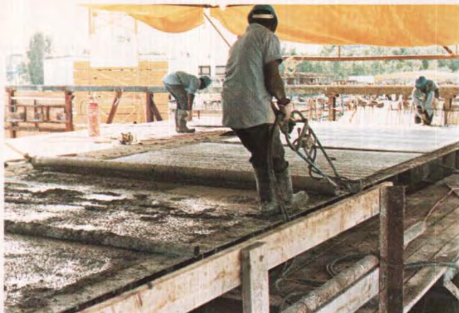
Fig. 16. Use of a rotary screed, followed by straightedge and light application of bull floats for a good finish.
