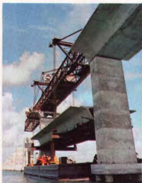
Fig. 13. Overhead gantry for span-by-span erection at Seven Mile Bridge.
