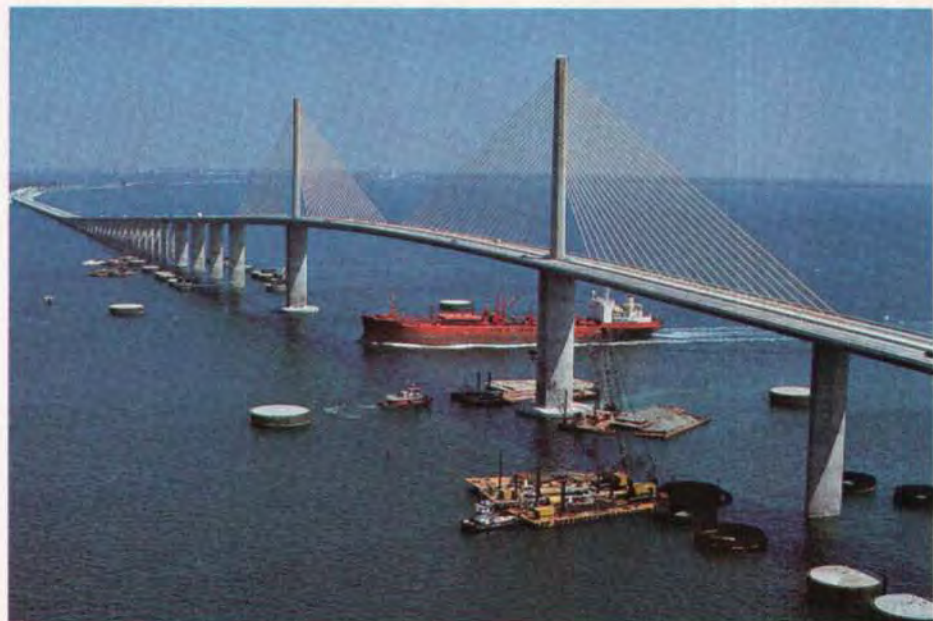
Fig. 9. Sunshine Skyway Bridge — A precast segmental, post-tensioned, cable stayed cantilever bridge with span-by-span high level approaches. (Courtesy of Figg and Muller Engineers Inc., Designer)
