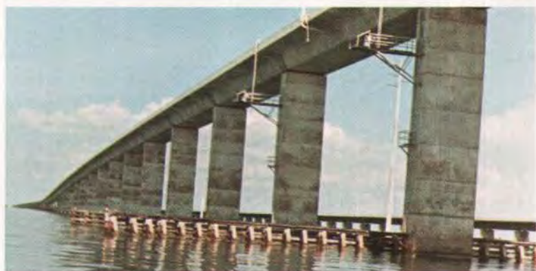
Fig. 10. Seven Mile Bridge — Precast vertically post-tensioned, segmental box piers.
