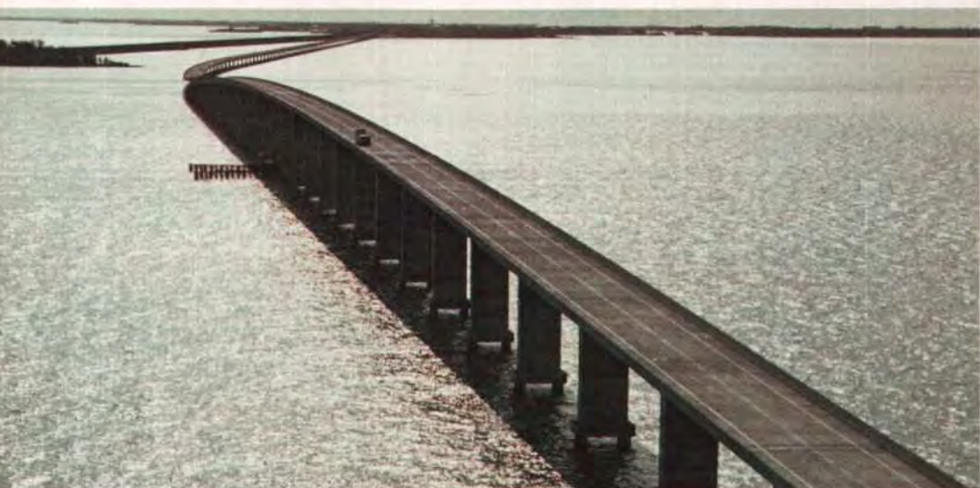
Fig. 2. Seven Mile Bridge — A precast segmental, post-tensioned, span-by-span structure. (Courtesy of Figg and Muller Engineers Inc., Designer)
