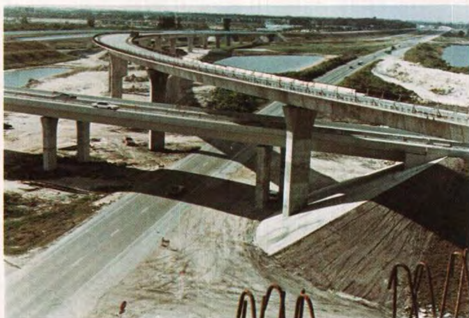
Fig. 19. I75/I595 Phase 2 project under construction.
