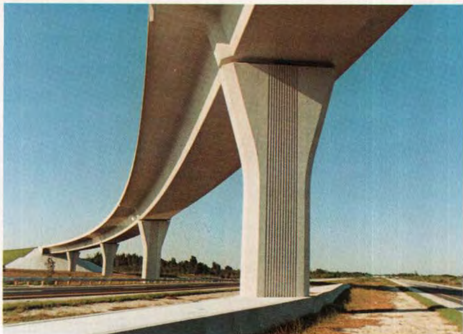
Fig. 3. Ramp I— A precast segmental, post-tensioned, balanced cantilever viaduct. (Courtesy of Beiswenger Hoch and Associates, Designer)
