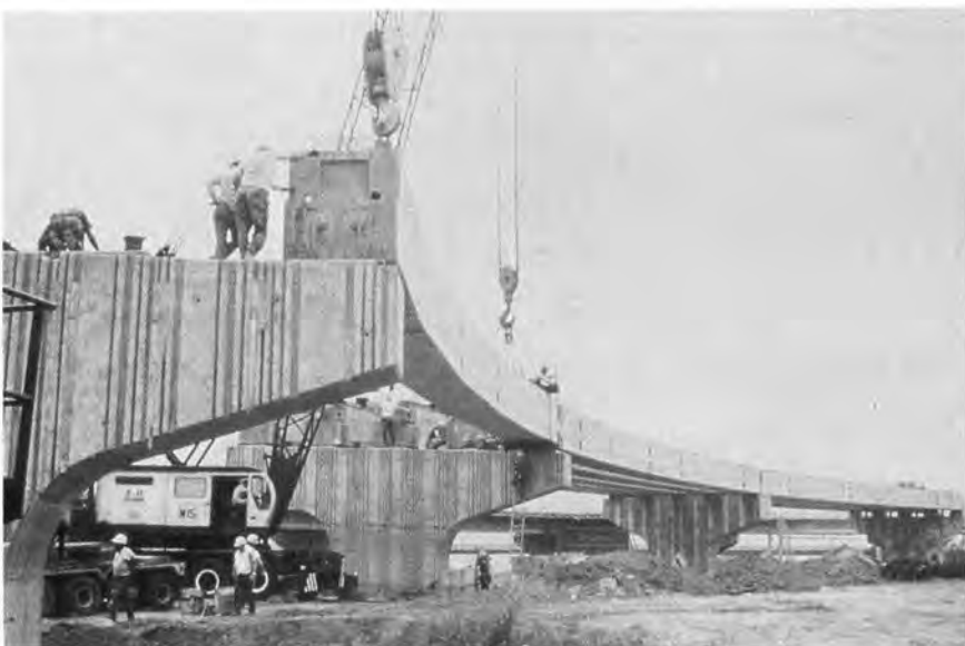
Fig. 7. Philadelphia Airport structure (Pennsylvania).
