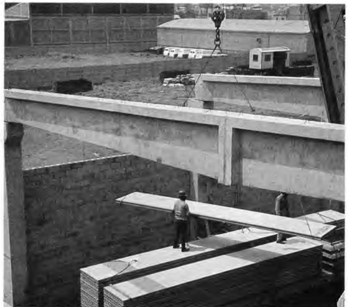
Fig. 12. Long span prestressed girders combined with hollow-core slabs (Mexico).
