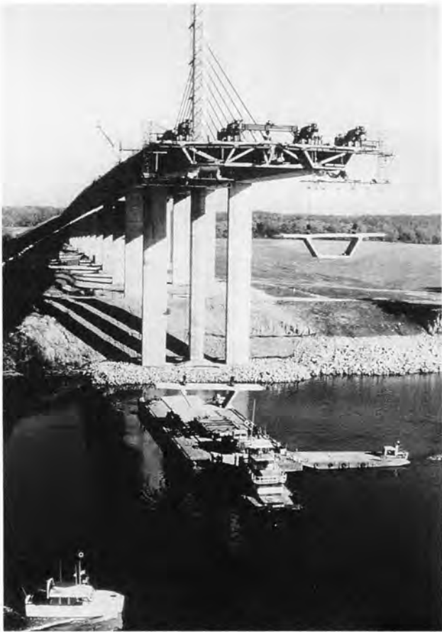
Fig. 6. James River Bridge (near Richmond, Virginia).
