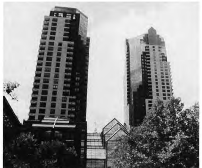
Fig. 13. High rise building in St. Paul, Minnesota, utilizing precast prestressed concrete components with the aid of post-tensioning.
