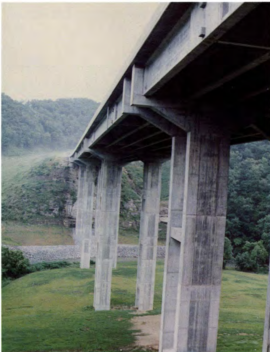
Fig. 9. Tall piers for high-level bridge.
