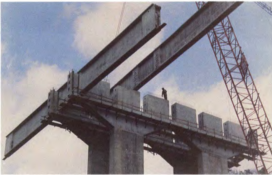
Fig. 4. Pier segments fit in pier cap slots.
