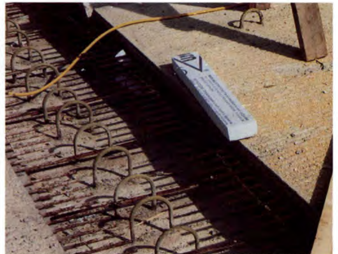
Fig. 21. High density foam strips used to support stay-in-place deck panels.
