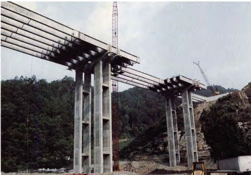
Fig. 6. Pier segments in place prior to receiving drop-in segments.
