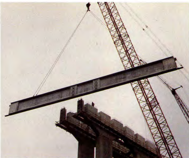
Fig. 16. Hoisting of 108 ft (33 m) bridge beam.
