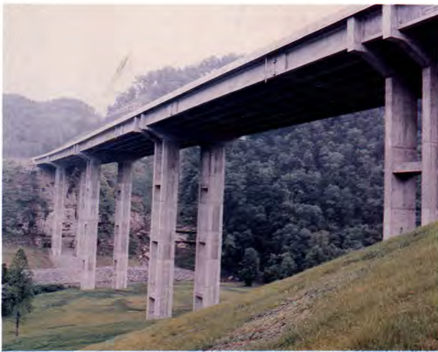
Fig. 25. Overall view of Shelby Creek Bridge, Pike County, Kentucky.
