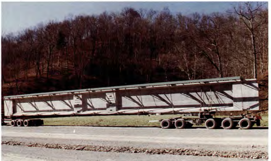
Fig. 13. Transportation of 108 ft (33 m) long bridge beam.
