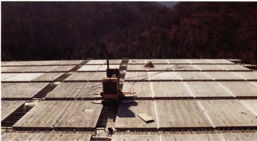
Fig. 23. Deck panels provide working surface until composite deck concrete is placed.
