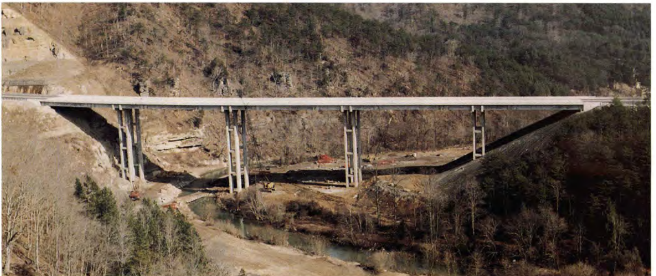
Fig. 24. Completed five-span highway bridge over Shelby Creek, Pike County, Kentucky.
