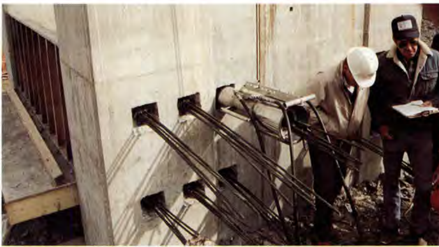
Fig. 10. Pier struts are post-tensioned to columns.
