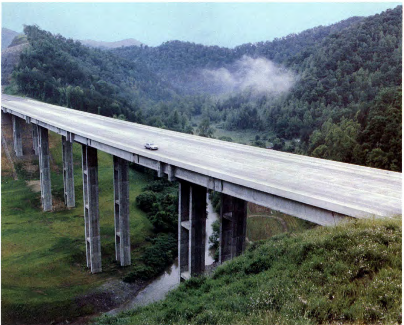
Fig. 1. Shelby Creek Bridge, Pike County, Kentucky.
