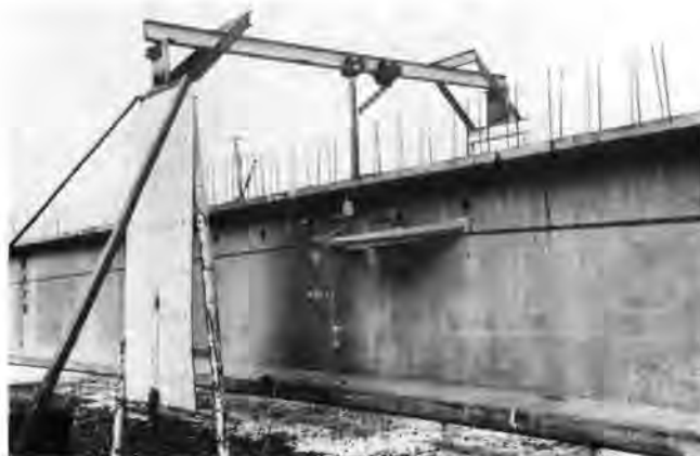
Fig. 24. King post bracing of a long prestressed concrete I-beam.
