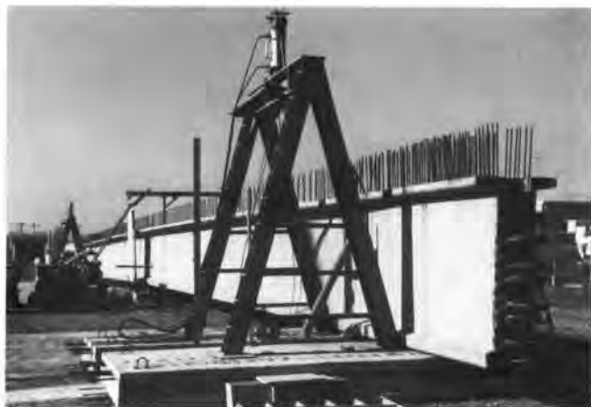
Fig. 5. Overall view of test setup for 149 ft (45.4 m) girder.
